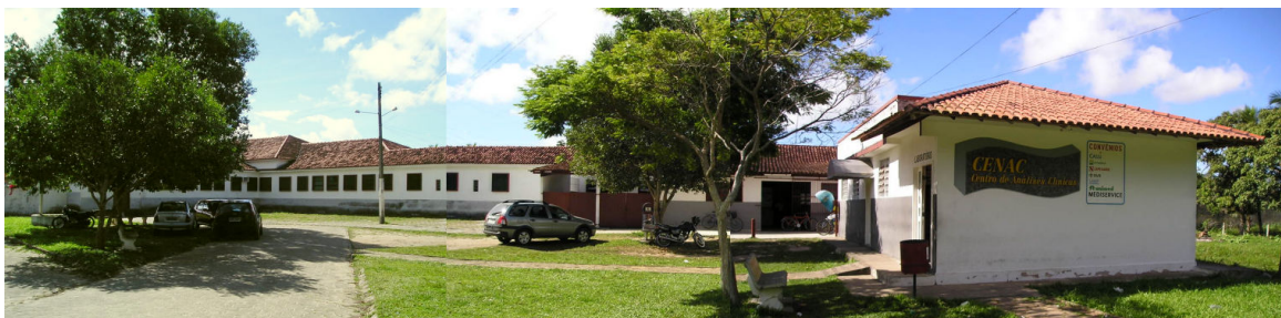
Figura 5.3.3-23 – Hospital Regional de Caravelas
