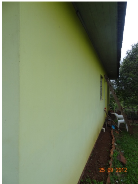
Fachada - Lateral (25/09/2012, 10:45h)
