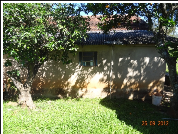
Fachada Lateral (25/09/2012, 14:28h)
