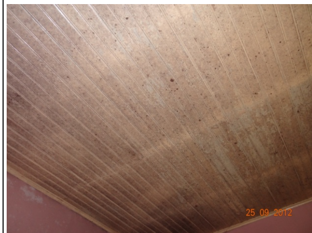
Forro madeira – Quarto (25/09/2012, 09:57h)
