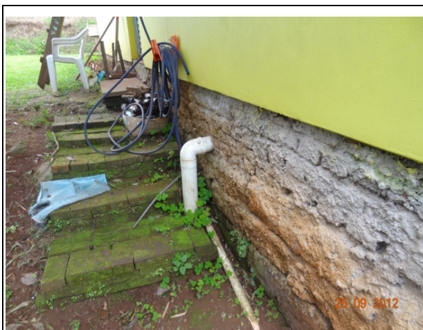
Fachada Fundos (25/09/2012, 10:43h)
