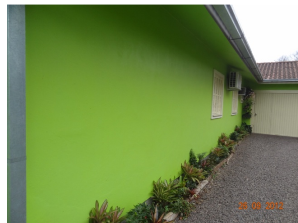
Fachada – Lateral (26/09/2012, 10:51h)
