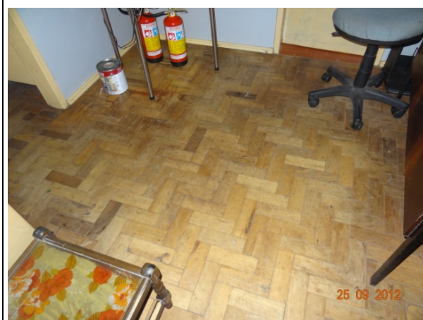
Piso – taco de madeira (25/09/2012, 09:53h)
