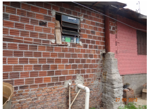
Fachada Lateral (27/09/2012, 14:32h)
