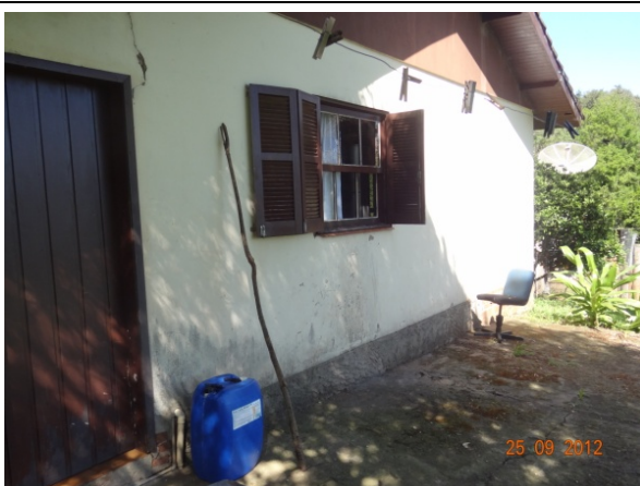
Fachada Fundos (25/09/2012, 14:29h)
