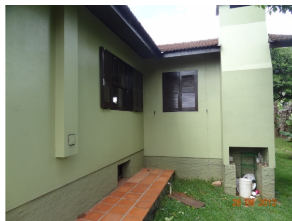
Fachada Lateral (26/09/2012, 11:21h)
