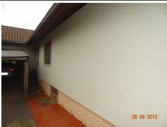
Fachada Lateral (26/09/2012, 10:38h)
