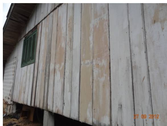
Fachada Lateral (27/09/2012, 14:48h)
