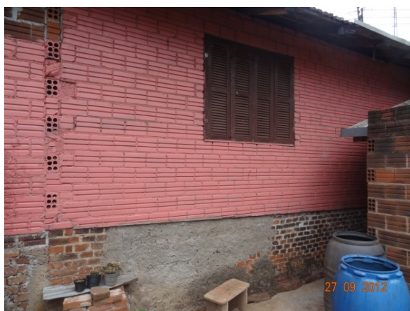
Fachada Lateral (27/09/2012, 14:32h)
