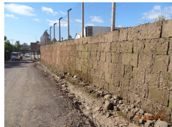
Muro – entrada Principal (26/09/2012, 15:52h)
