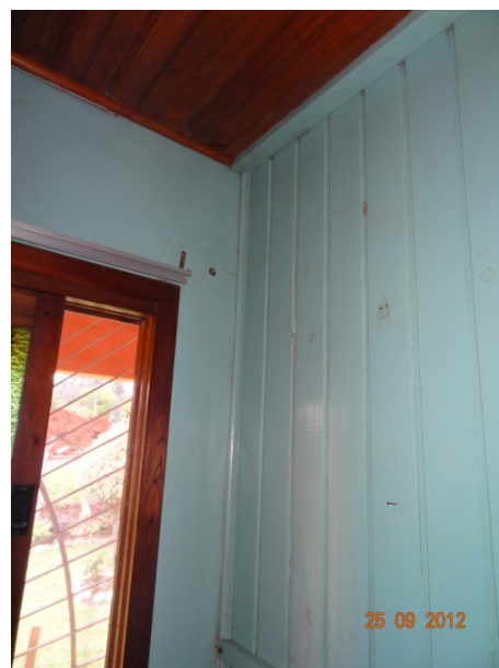
Paredes interna de madeira (25/09/2012,09:34h)
