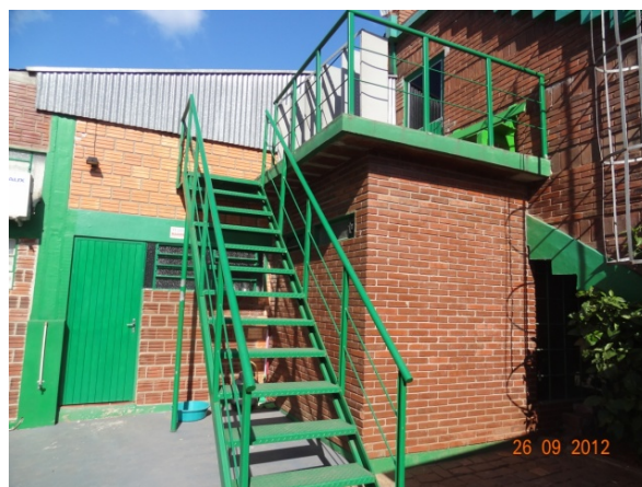
Fachada Lateral (26/09/2012, 15:35h)
