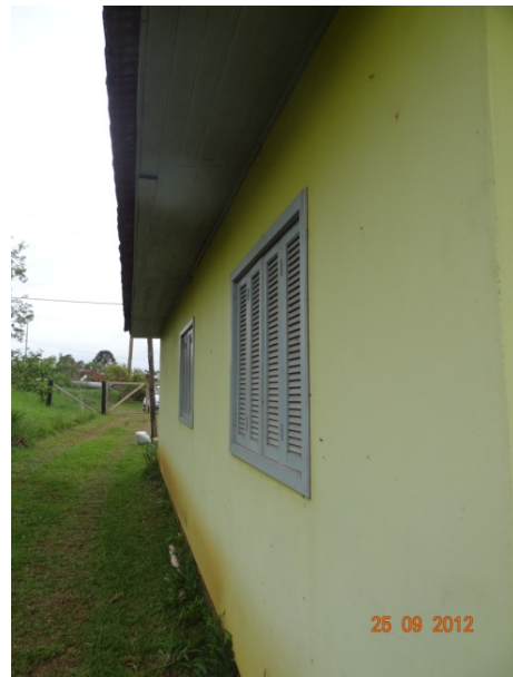
Fachada – Lateral (25/09/2012, 10:45h)
