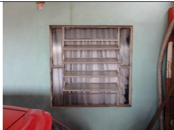
Fachada (DSC03619, 23/02/2011, 09:51h)
