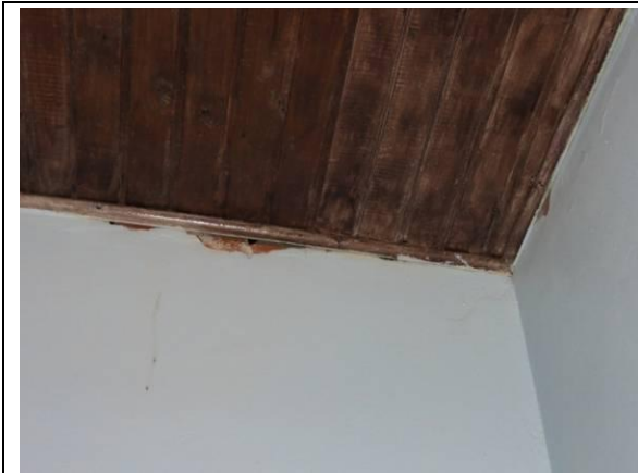
WC 1 e WC 2 (DSC04607, 24/02/2011, 10:10h)
