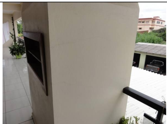
Piso Superior – Area (DSC03996, 23/02/2011, 11:23h)
