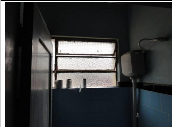
WC 1 e WC 2 (DSC04599, 24/02/2011, 10:09h)
