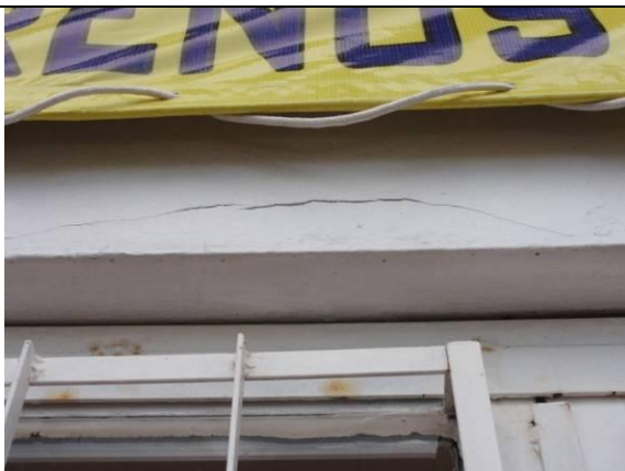
Fachada (DSC04345, 24/02/2011, 09:16h)
