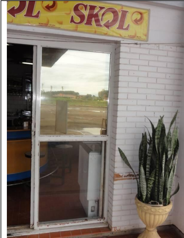
Fachada (DSC04703, 24/02/2011, 11:06h)
