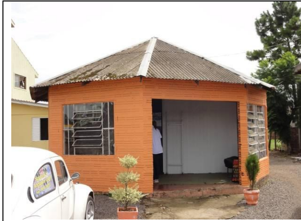
Fachada (DSC03682, 23/02/2011, 10:06h)
