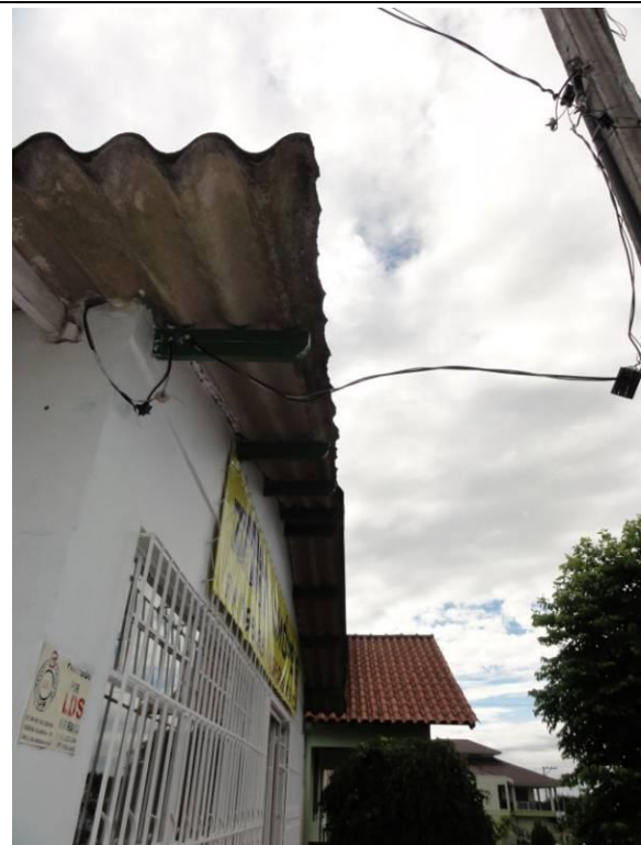
Fachada (DSC04380, 24/02/2011, 09:21h)
