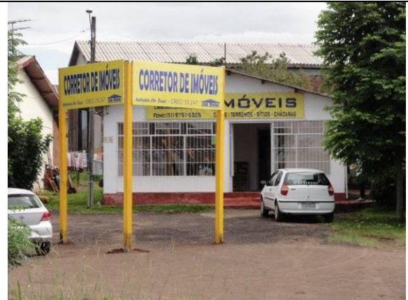
Fachada (DSC04326, 24/02/2011, 09:12h)
