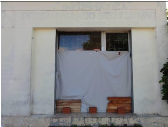
Fachada (DSC04479, 24/02/2011, 09:46h)
