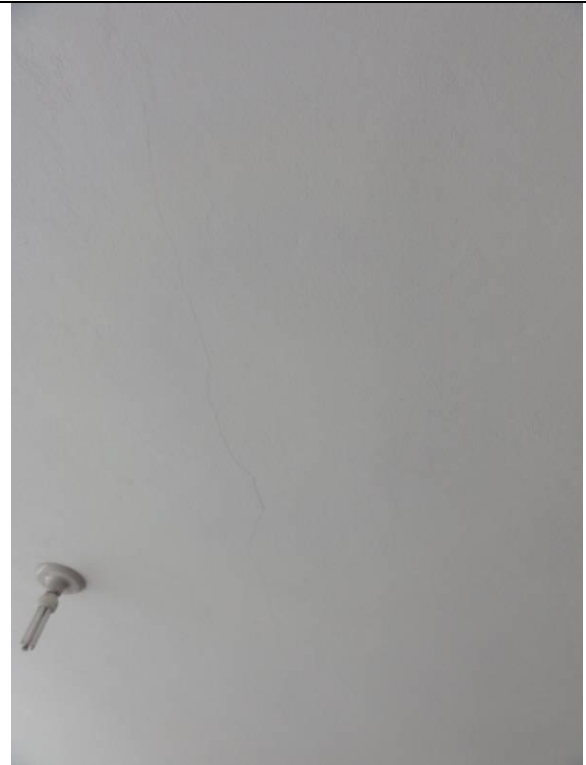
Piso Superior – Area (DSC04010, 23/02/2011, 11:26h)
