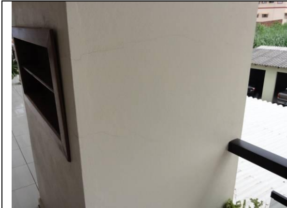
Piso Superior – Area (DSC03997, 23/02/2011, 11:23h)
