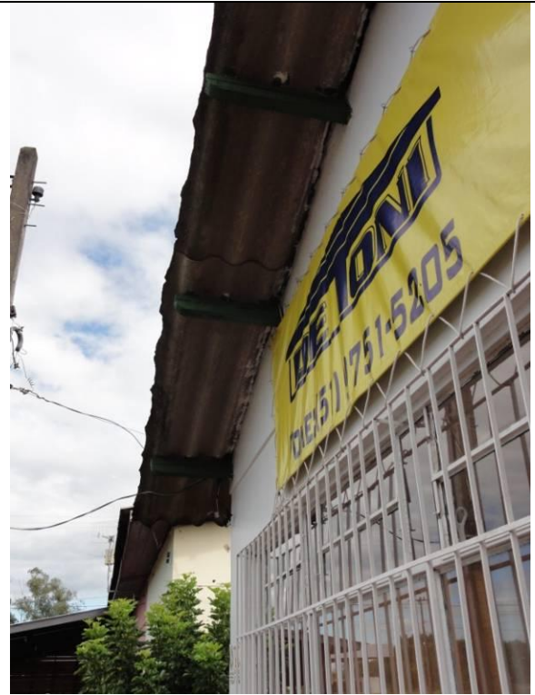
Fachada – Marquise (DSC04338, 24/02/2011, 09:15h)
