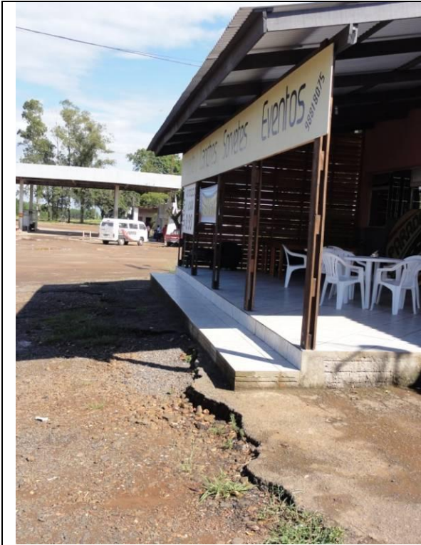
Fachada (DSC04477, 24/02/2011, 09:45h)
