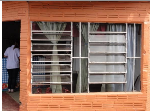
Fachada (DSC03684, 23/02/2011, 10:06h)
