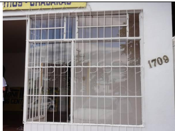
Fachada (DSC04346, 24/02/2011, 09:17h)
