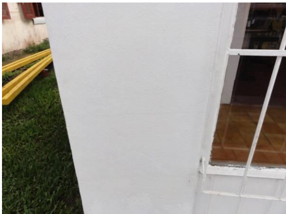
Fachada (DSC04341, 24/02/2011, 09:15h)
