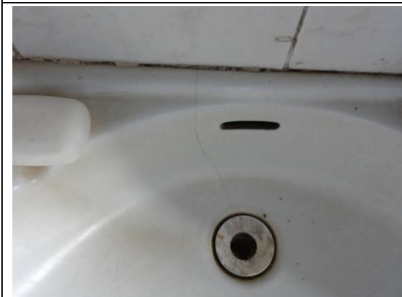
WC 1 e WC 2 (DSC04605, 24/02/2011, 10:09h)
