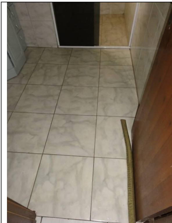
Piso Superior – WC (DSC04047, 23/02/2011, 11:36h)
