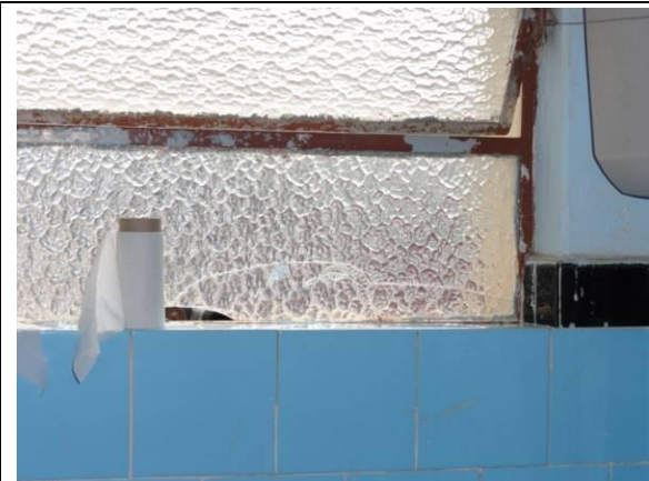
WC 1 e WC 2 (DSC04600, 24/02/2011, 10:09h)
