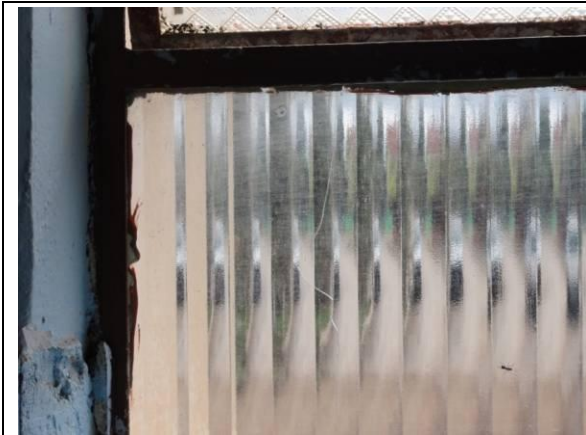
WC 1 e WC 2 (DSC04603, 24/02/2011, 10:09h)
