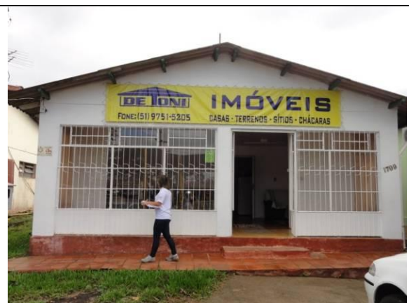
Fachada (DSC04328, 24/02/2011, 09:13h)
