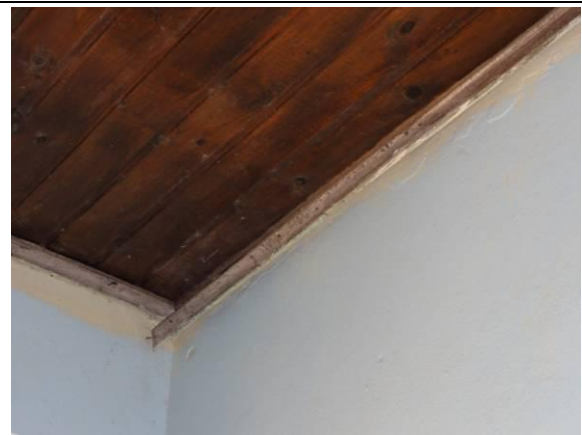
WC 1 e WC 2 (DSC04612, 24/02/2011, 10:11h)
