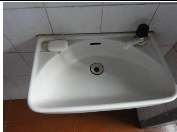
WC 1 e WC 2 (DSC04604, 24/02/2011, 10:09h)
