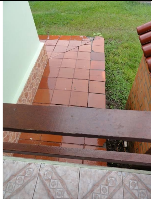
Fachada – Area (DSC04252, 23/02/2011, 17:16h)
