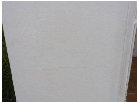
Fachada (DSC04342, 24/02/2011, 09:15h)
