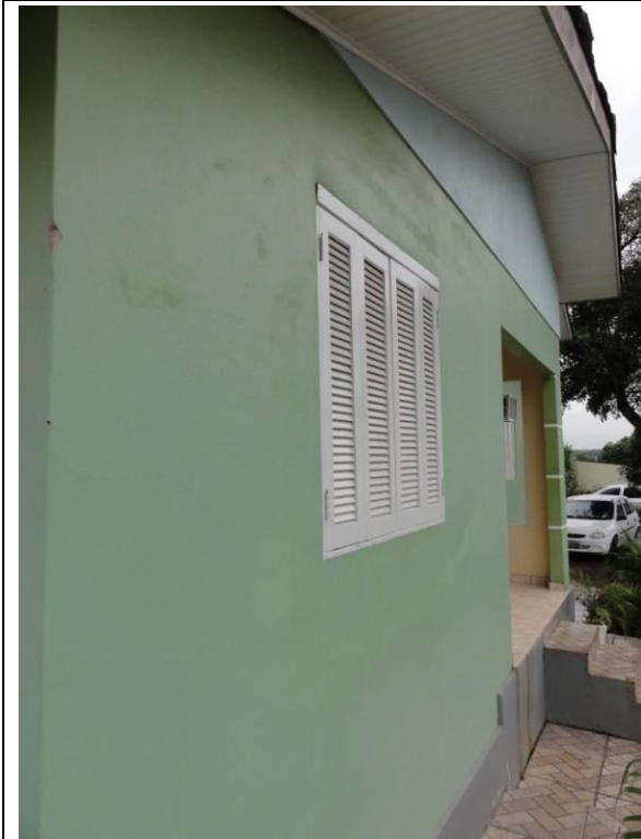
Fachada (DSC04164, 23/02/2011, 16:50h)
