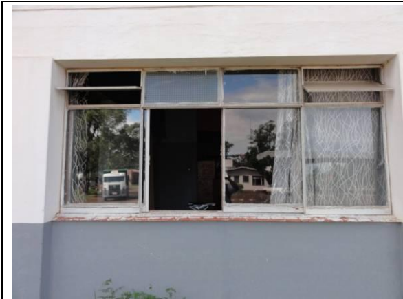
Parede B (DSC04506, 24/02/2011, 09:51h)
