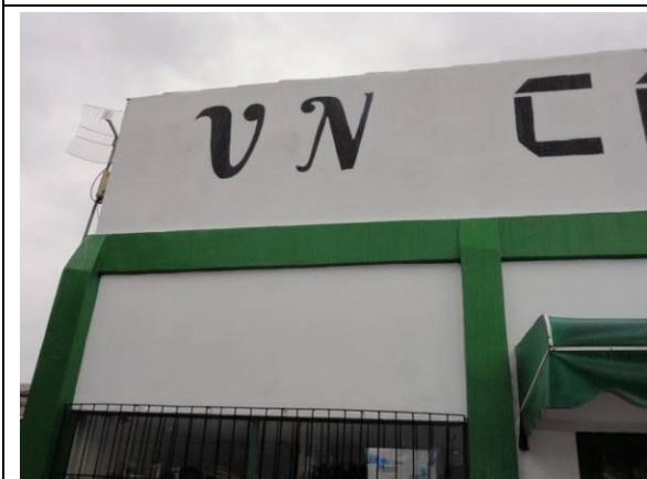
Fachada (DSC04098, 23/02/2011, 16:34h)
