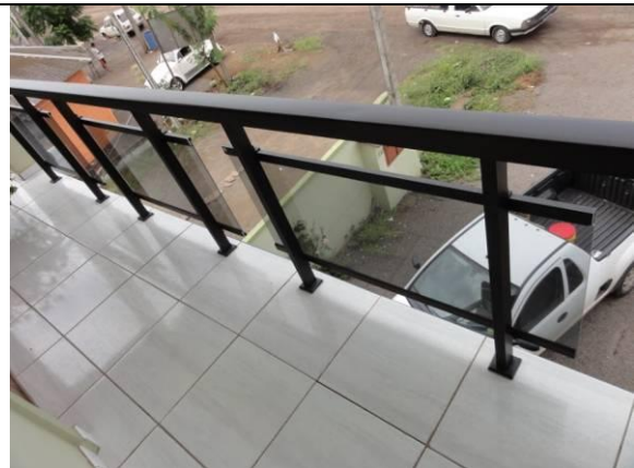
Piso Superior - Sacada (DSC03968, 23/02/2011, 11:19h)
