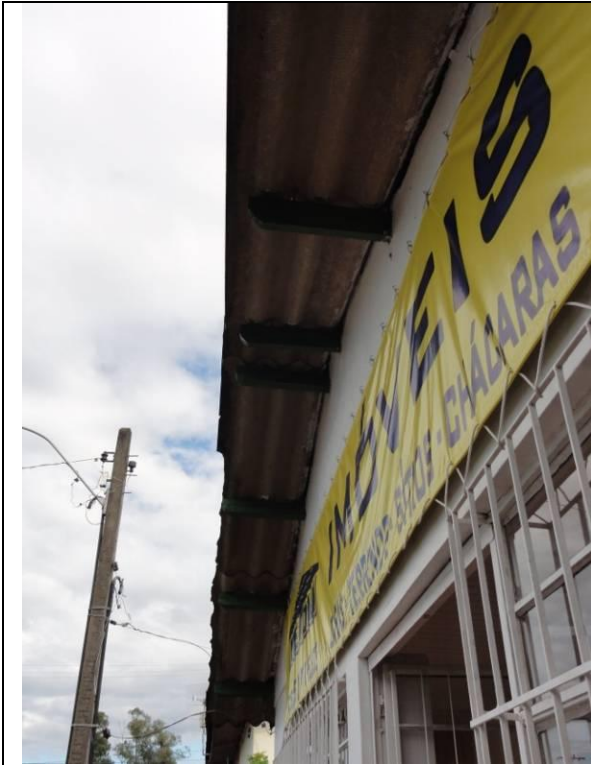
Fachada – Marquise (DSC04337, 24/02/2011, 09:14h)
