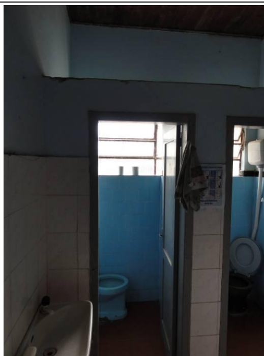
WC 1 e WC 2 (DSC04598, 24/02/2011, 10:09h)
