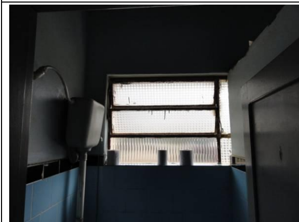
WC 1 e WC 2 (DSC04601, 24/02/2011, 10:09h)
