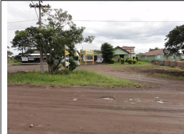
Fachada (DSC04325, 24/02/2011, 09:12h)
