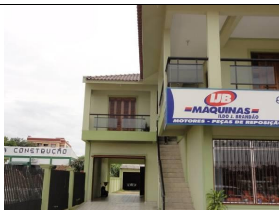
Fachada (DSC03914, 23/02/2011, 11:11h)
