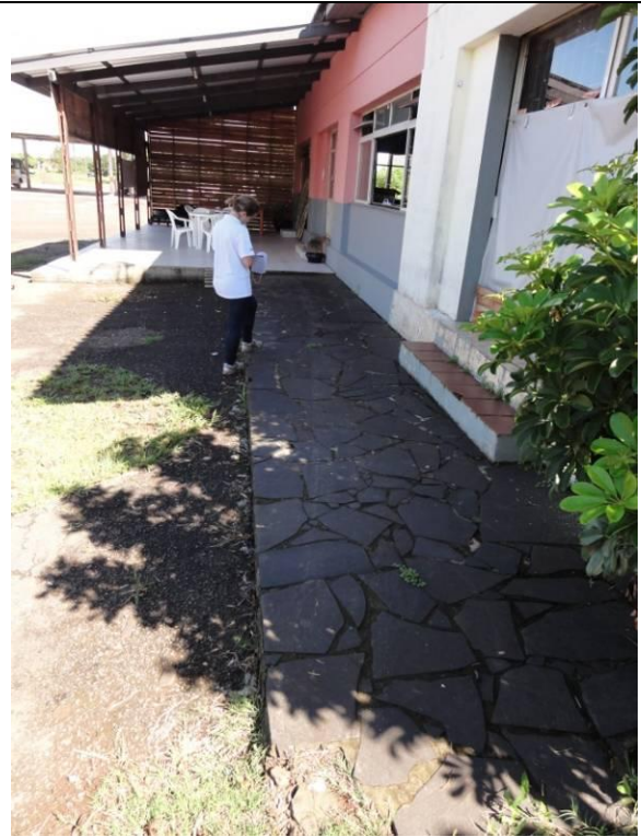
Fachada (DSC044780, 24/02/2011, 09:46h)
