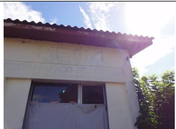
Fachada (DSC04480, 24/02/2011, 09:46h)
