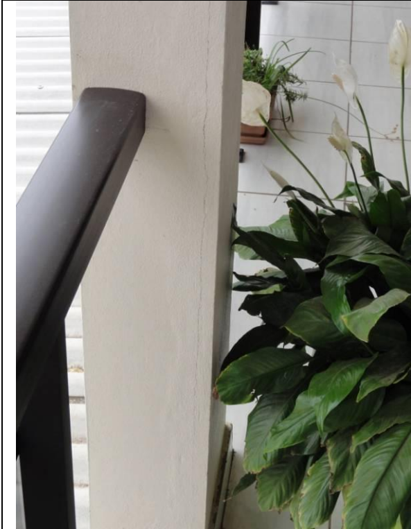
Piso Superior – Area (DSC03989, 23/02/2011, 11:22h)
