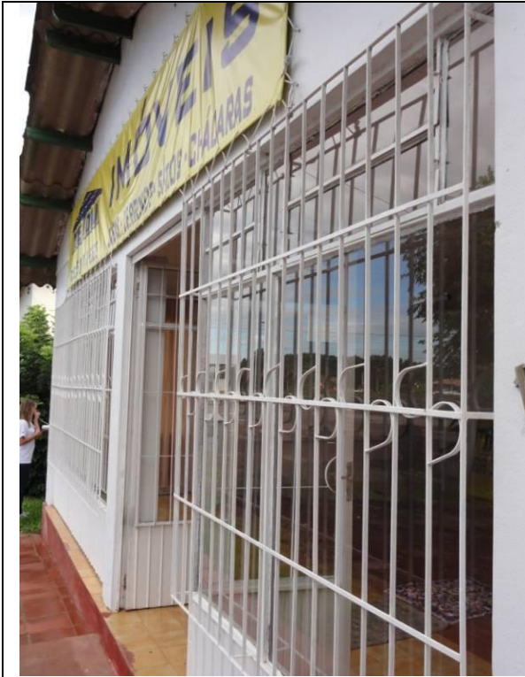
Fachada (DSC04335, 24/02/2011, 09:14h)
