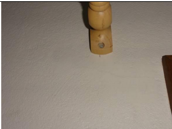
Piso Superior – Quarto 5 (DSC04057, 23/02/2011, 11:38h)
