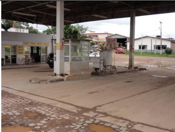
Fachada (DSC04695, 24/02/2011, 11:05h)
