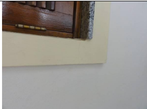
Piso Superior – Area (DSC04004, 23/02/2011, 11:24h)
