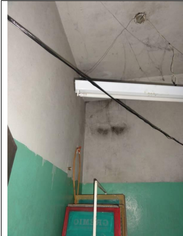
Piso Inferior – Loja – WC 1 (DSC03426, 23/02/2011, 09:05h)
