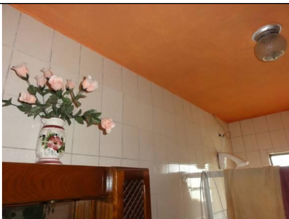
Piso superior – WC 1 (DSC02374, 21/02/2011, 16:14h)
