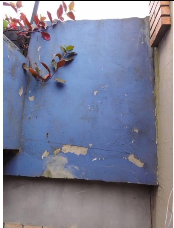
Piso Superior – Sacada (DSC03605, 23/02/2011, 09:40h)
