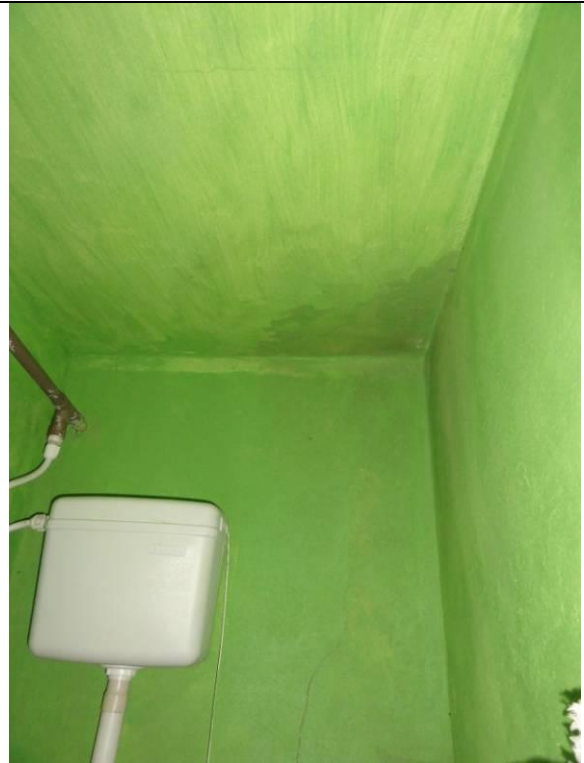
Piso superior - WC 2 (DSC02455, 21/02/2011, 16:35h)
