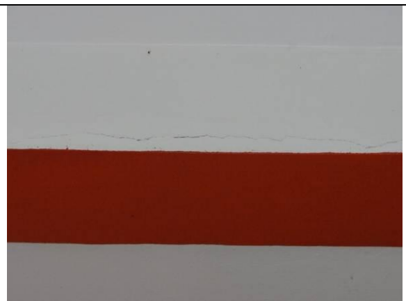
Piso inferior – Hall – Teto (DSC02820, 22/02/2011, 09:41h)
