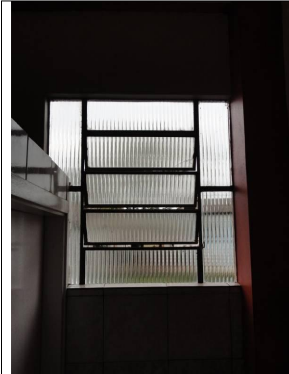
Piso inferior – WC – Janela rachado (DSC02827, 22/02/2011, 09:43h)
