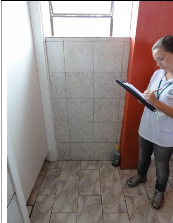
Piso inferior – WC (DSC02829, 22/02/2011, 09:44h)
