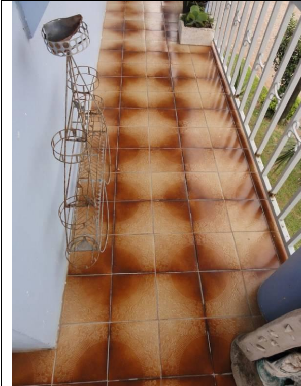
Piso superior – Sacada (DSC02336, 21/02/2011, 16:06h)
