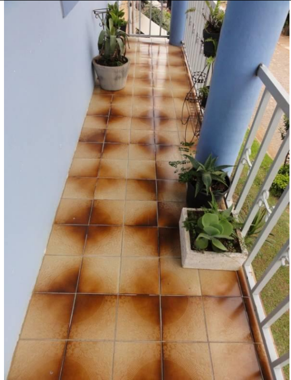
Piso superior – Sacada (DSC02337, 21/02/2011, 16:07h)
