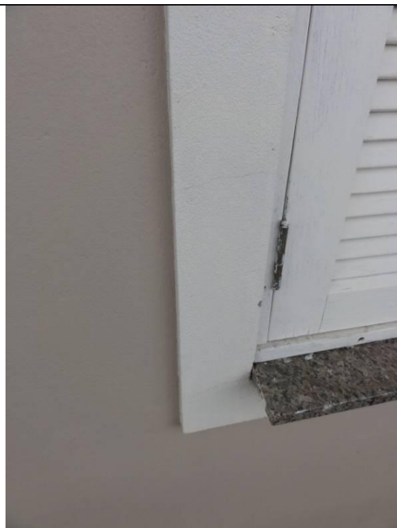
Piso superior – Sacada (DSC02963, 22/02/2011, 10:16h)
