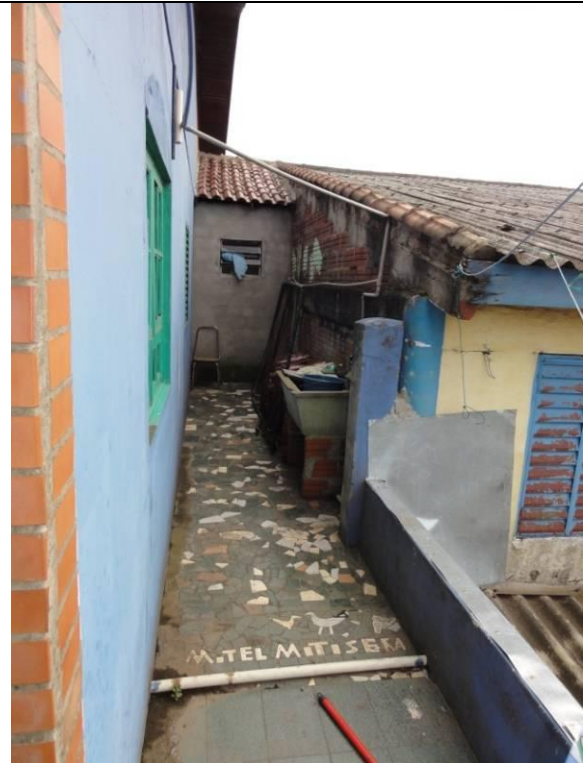
Piso Superior – Sacada (DSC03593, 23/02/2011, 09:39h)
