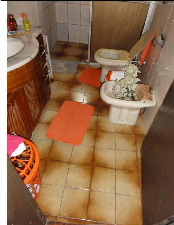
Piso superior – WC 1 (DSC02382, 21/02/2011, 16:15h)
