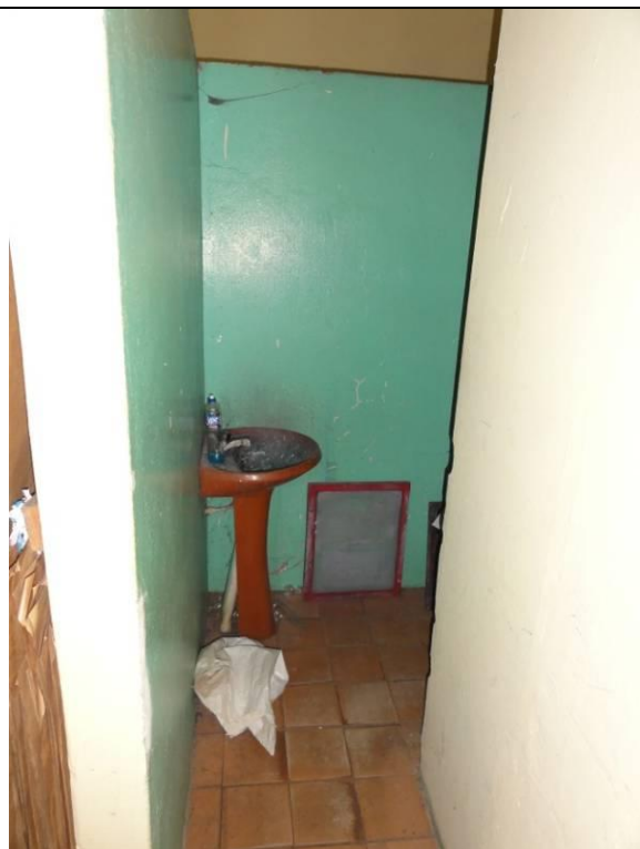
Piso Inferior – Loja – WC 1 (DSC03423, 23/02/2011, 09:04h)
