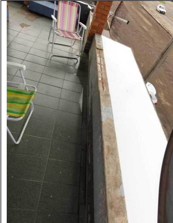
Piso Superior – Sacada (DSC03600, 23/02/2011, 09:39h)
