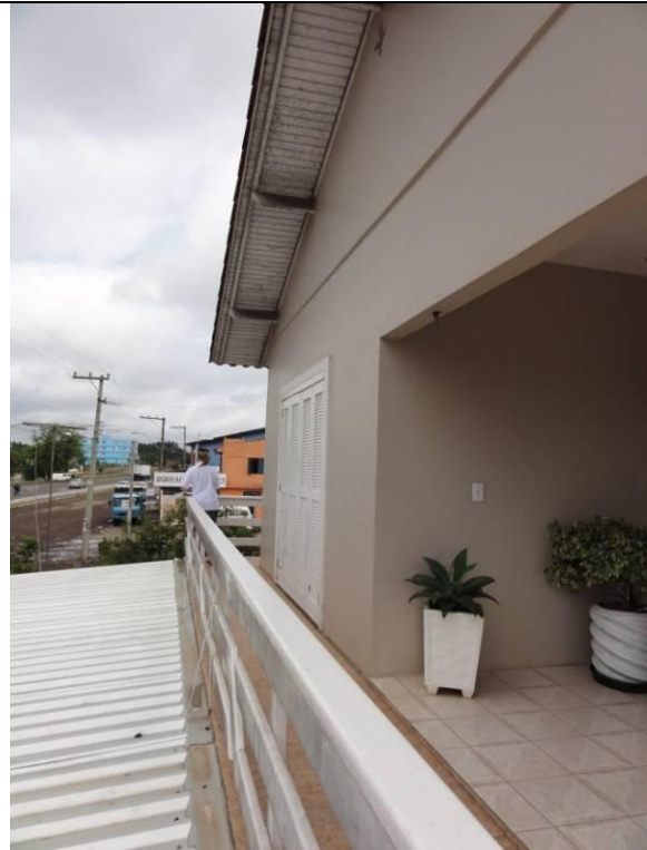
Piso superior - Sacada (DSC02893, 22/02/2011, 10:05h)
