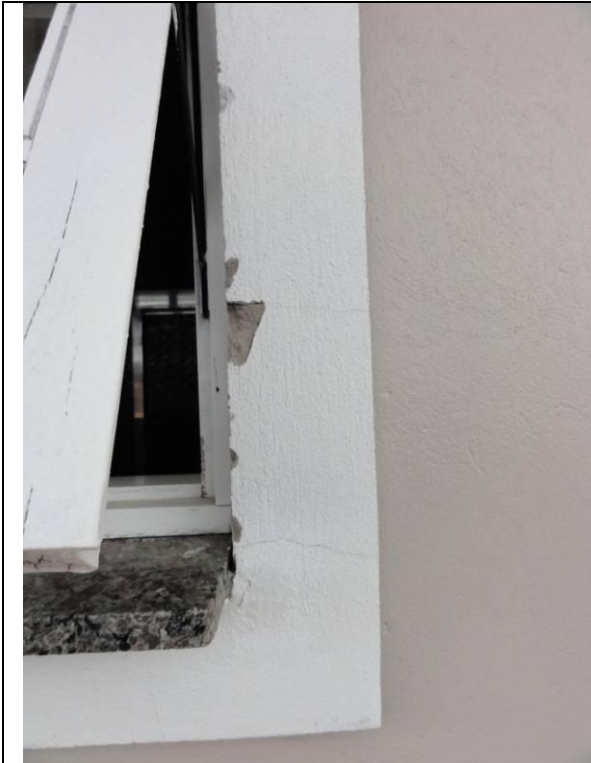
Piso superior – Sacada (DSC02960, 22/02/2011, 10:16h)
