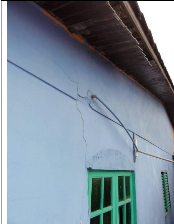
Piso Superior - Sacada (DSC03572, 23/02/2011, 09:36h)
