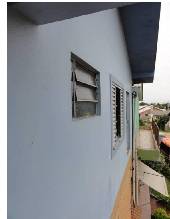
Piso superior (DSC02346, 21/02/2011, 16:08h)
