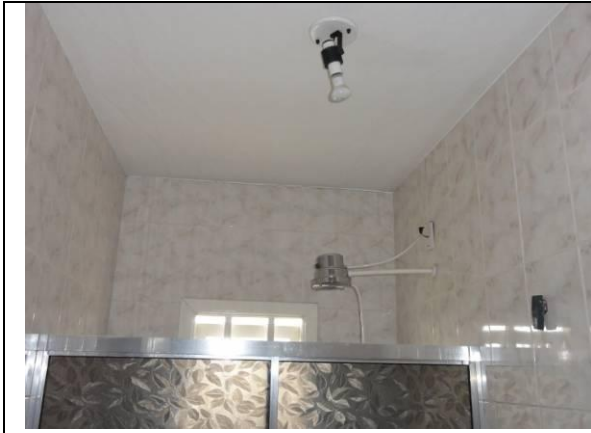
Piso superior – WC 1 (DSC02982, 22/02/2011, 10:21h)
