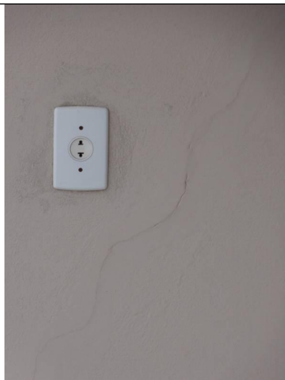
Piso superior – Sacada (DSC02923, 22/02/2011, 10:09h)
