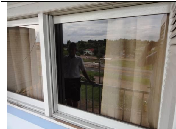
Piso superior – Janela (DSC02326, 21/02/2011, 16:05h)
