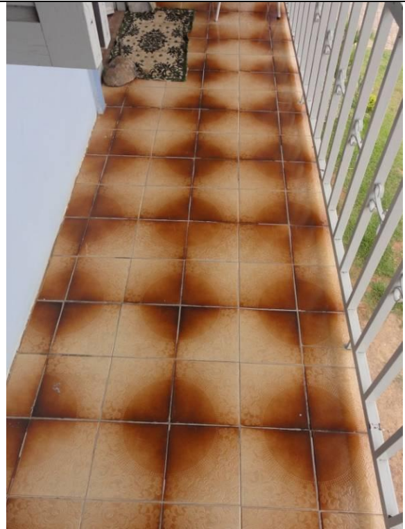
Piso superior – Sacada (DSC02321, 21/02/2011, 16:04h)
