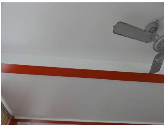
Piso inferior – Hall – Teto (DSC02819, 22/02/2011, 09:41h)
