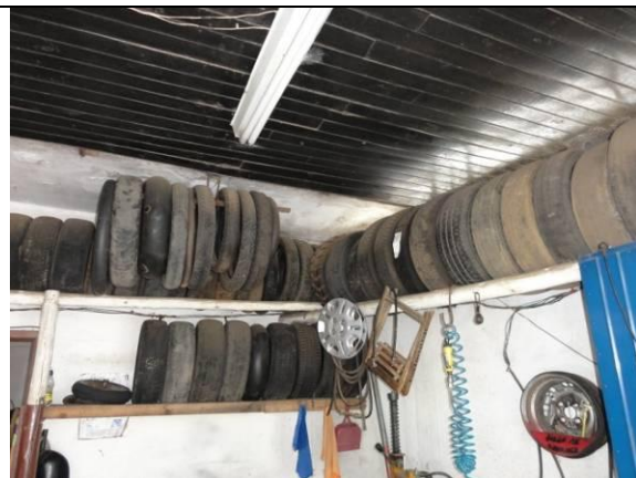
Piso Inferior - Borracharia (DSC03045, 22/02/2011, 10:58h)
