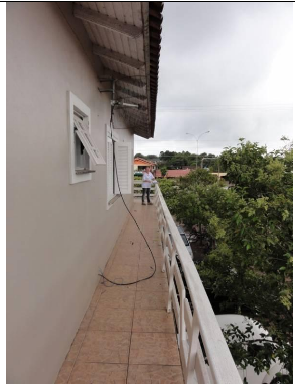
Piso superior – Sacada (DSC02951, 22/02/2011, 10:15h)
