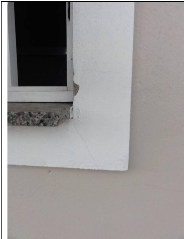
Piso superior – Sacada (DSC02940, 22/02/2011, 10:13h)
