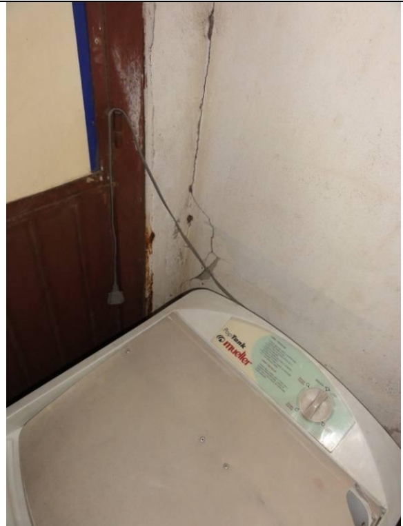
Piso Inferior – Borracharia (DSC03071, 22/02/2011, 11:03h)
