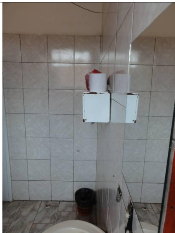
Piso inferior – WC (DSC02832, 22/02/2011, 09:45h)
