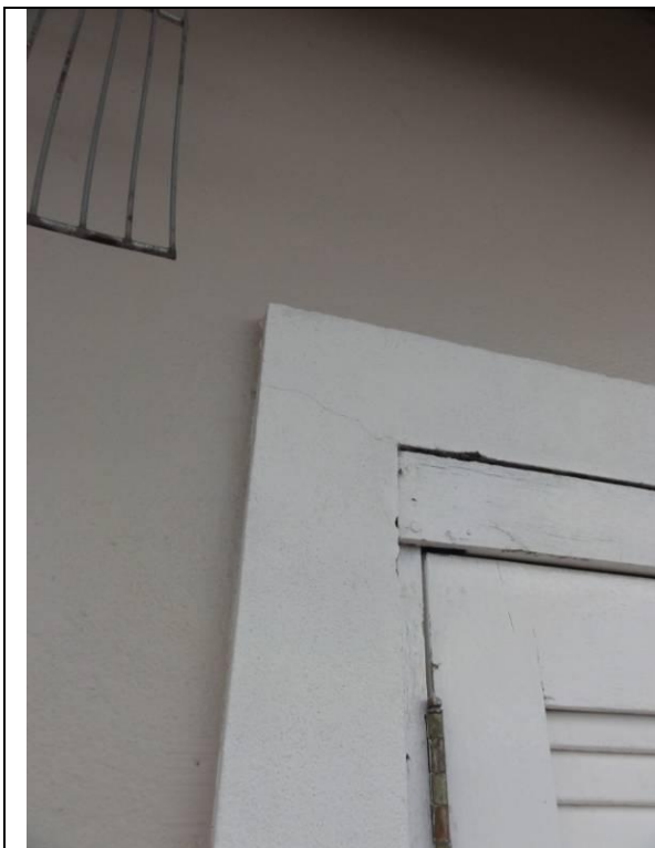
Piso superior – Sacada (DSC02962, 22/02/2011, 10:16h)
