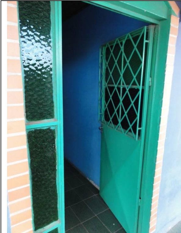
Piso Superior - Sacada (DSC03554, 23/02/2011, 09:34h)
