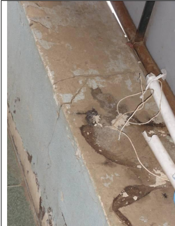
Piso Superior - Sacada (DSC03548, 23/02/2011, 09:33h)
