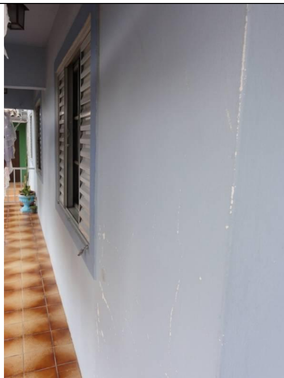
Piso superior – Sacada (DSC02319, 21/02/2011, 16:04h)
