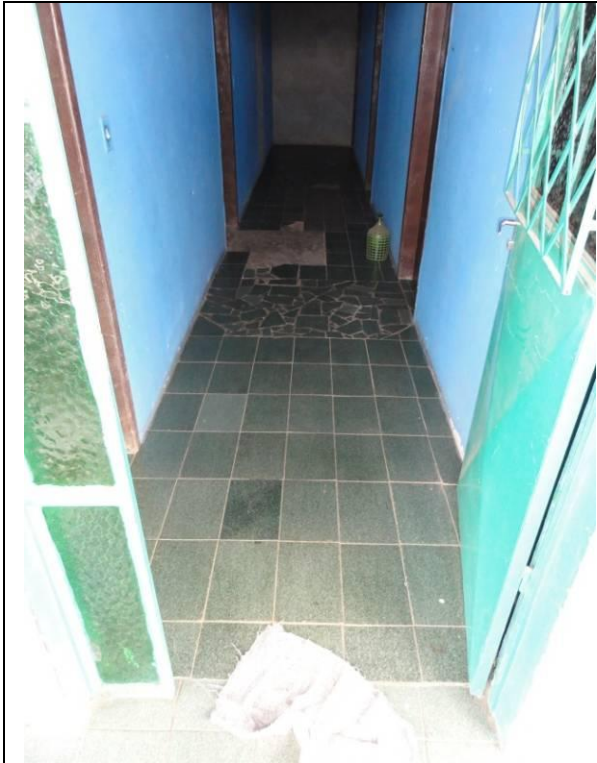
(Piso Superior – Sacada (DSC03598, 23/02/2011, 09:39h)
