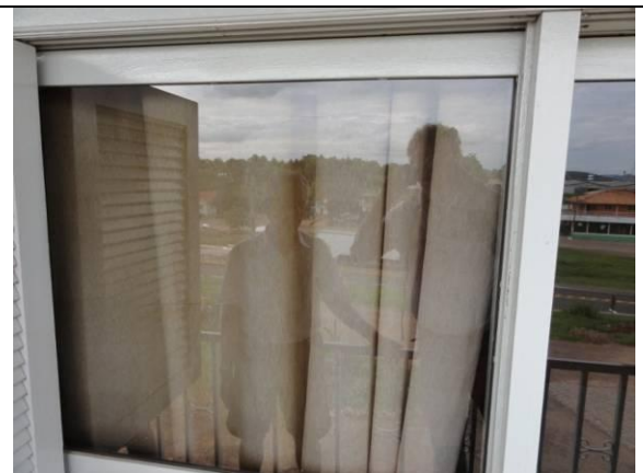
Piso superior – Janela (DSC02327, 21/02/2011, 16:05h)
