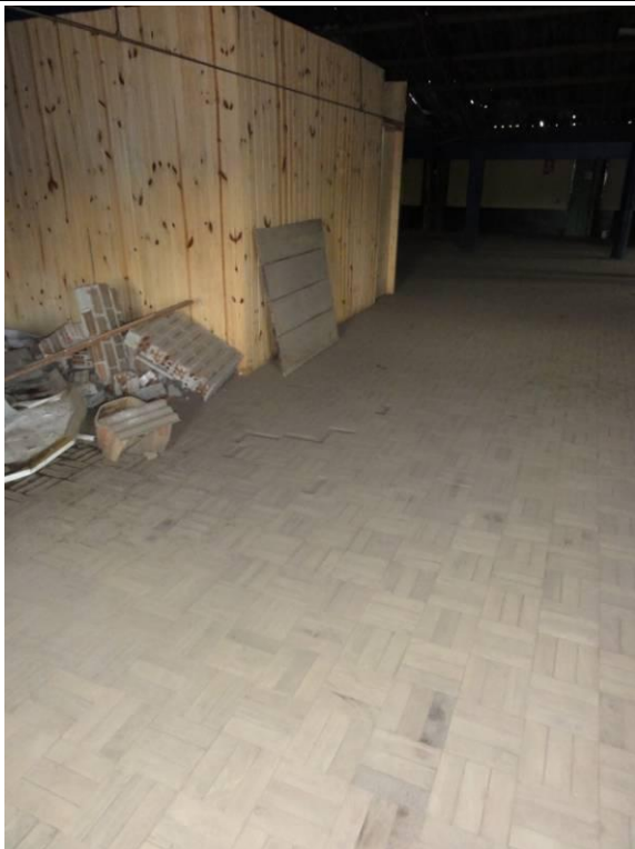
Piso superior (DSC03280, 22/02/2011, 17:06h)
