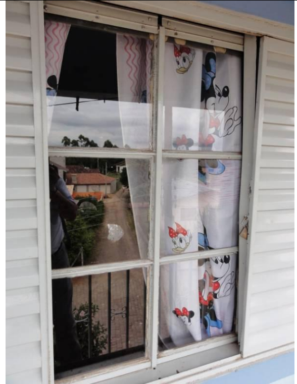
Piso superior – Sacada (DSC02339, 21/02/2011, 16:07h)
