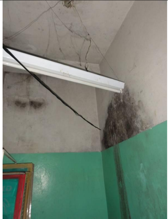
Piso Inferior – Loja – WC 1 (DSC03425, 23/02/2011, 09:05h)
