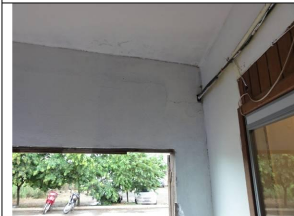
Piso Inferior – Fábrica (DSC03129, 22/02/2011, 16:36h)
