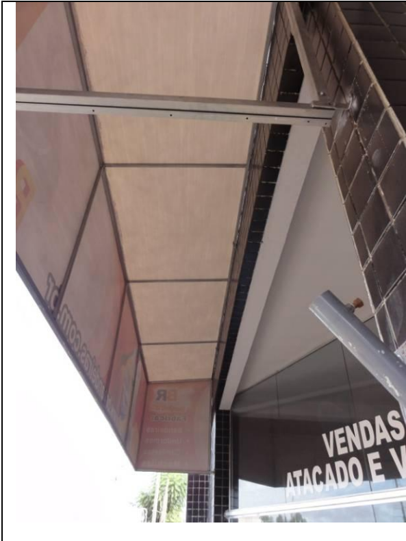
Fachada – Toldo (DSC03372, 23/02/2011, 08:55h)
