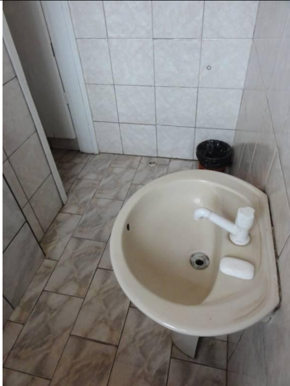
Piso inferior – WC (DSC02833, 22/02/2011, 09:45h)
