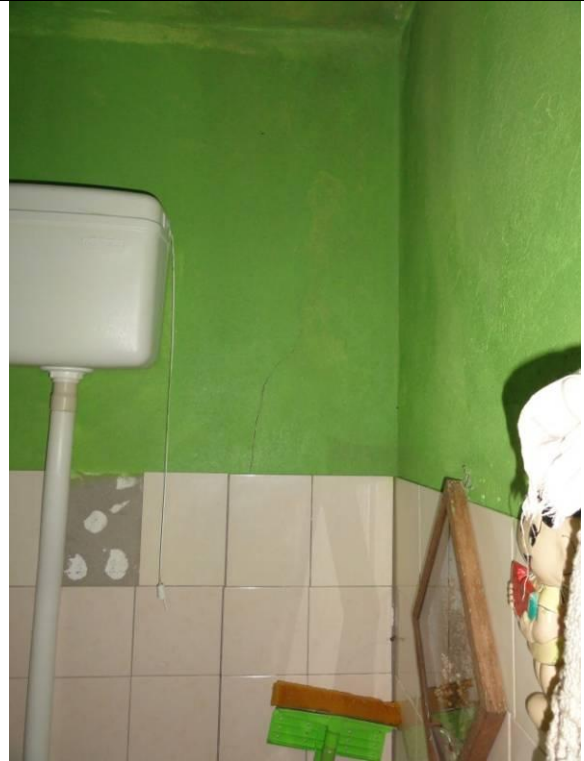
Piso superior - WC 2 (DSC02453, 21/02/2011, 16:35h)
