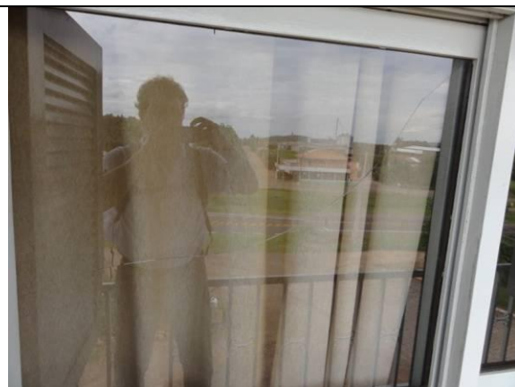
Piso superior – Janela (DSC02329, 21/02/2011, 16:05h)
