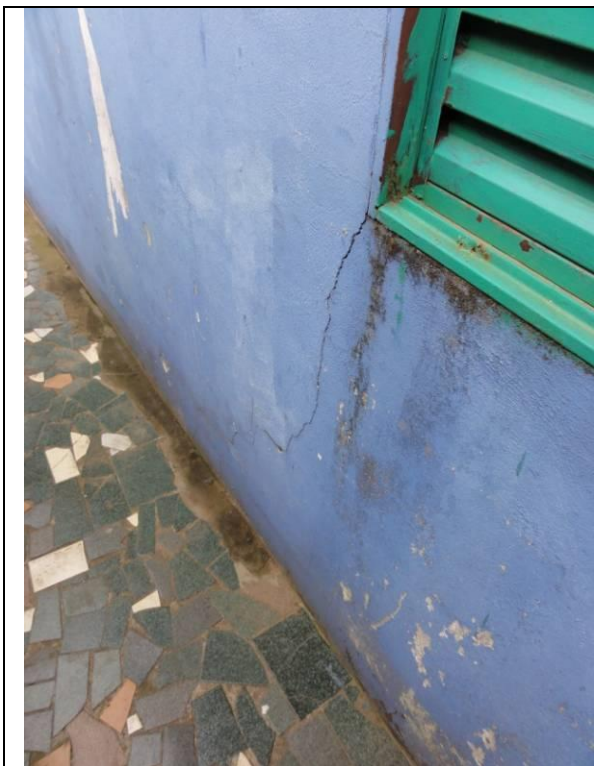
Piso Superior – Sacada (DSC03590, 23/02/2011, 09:38h)
