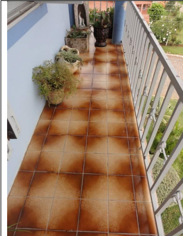
Piso superior – Sacada (DSC02324, 21/02/2011, 16:04h)
