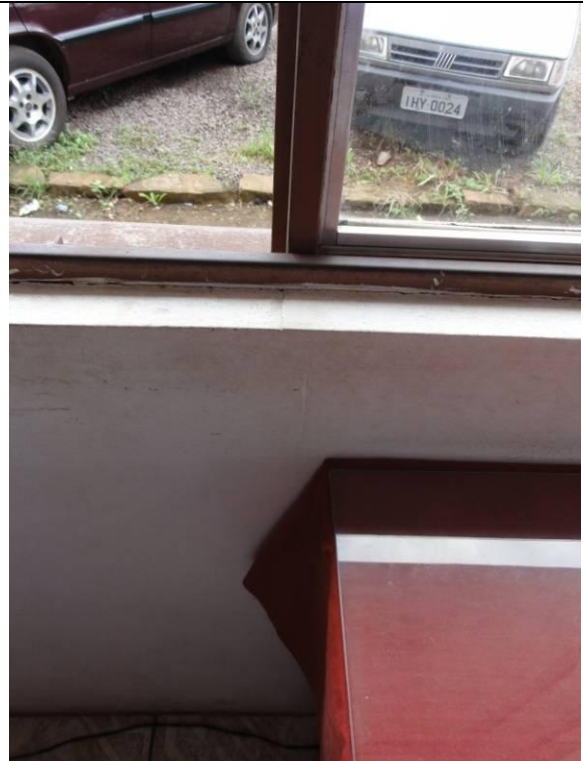
Piso inferior – Hall (DSC02822, 22/02/2011, 09:42h)
