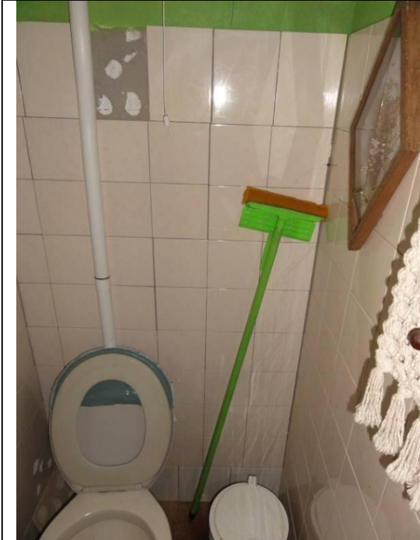
Piso superior - WC 2 (DSC02452, 21/02/2011, 16:35h)
