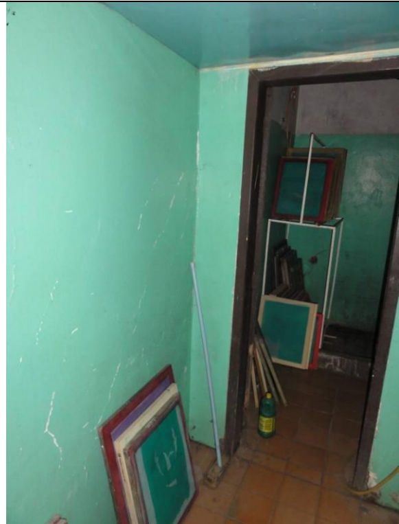
Piso Inferior – Loja – WC 1 (DSC03427, 23/02/2011, 09:05h)
