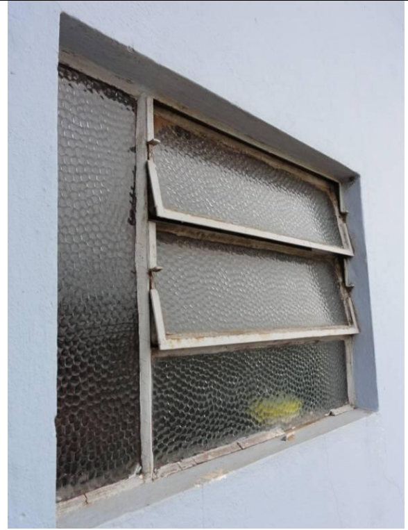
Piso superior (DSC02349, 21/02/2011, 16:08h)
