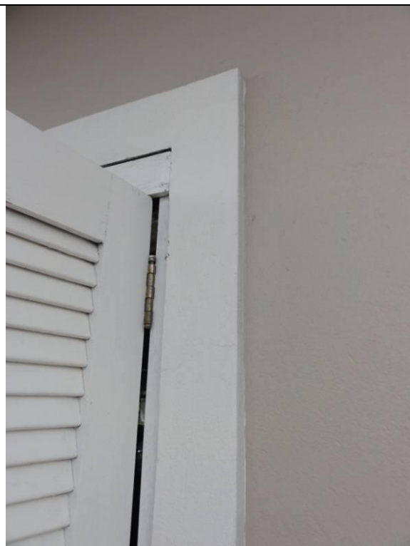
Piso superior – Sacada (DSC02965, 22/02/2011, 10:16h)
