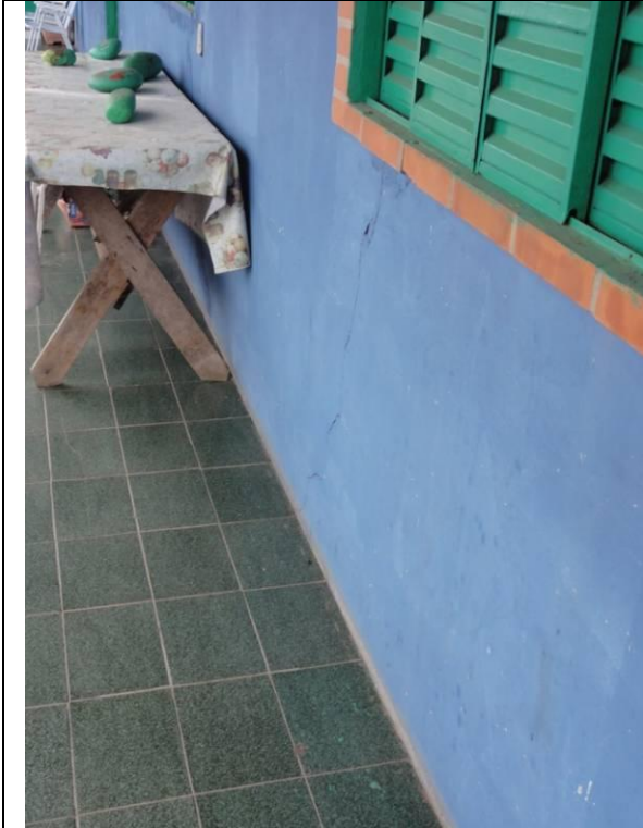
Piso Superior – Sacada (DSC03602, 23/02/2011, 09:40h)
