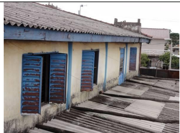
Piso Superior – Sacada (DSC03595, 23/02/2011, 09:39h)
