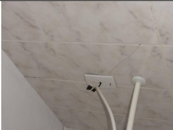
Piso superior – WC 1 (DSC02984, 22/02/2011, 10:22h)
