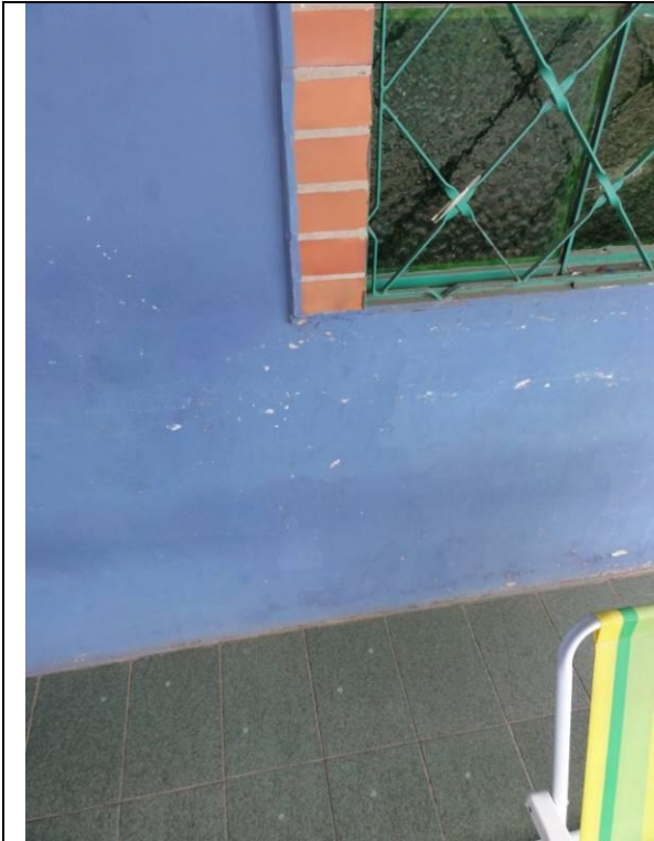
Piso Superior - Sacada (DSC03558, 23/02/2011, 09:34h)
