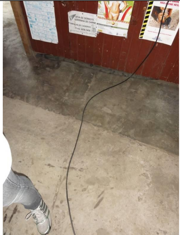
Piso Inferior – Borracharia (DSC03075, 22/02/2011, 11:04h)
