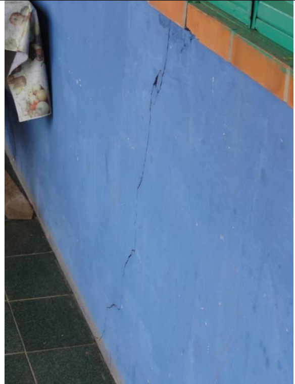
Piso Superior – Sacada (DSC03603, 23/02/2011, 09:40h)
