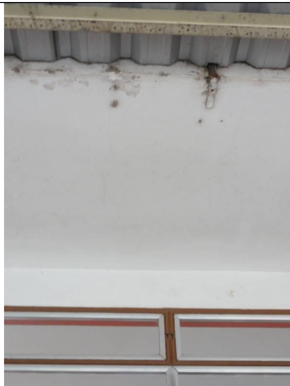
Piso inferior – Hall – Teto (DSC02810, 22/02/2011, 09:39h)
