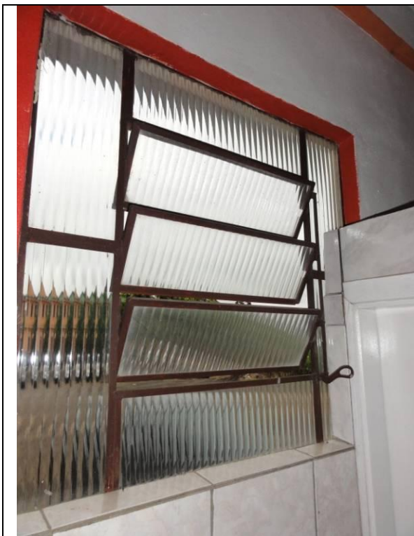
Piso inferior – WC (DSC02831, 22/02/2011, 09:44h)
