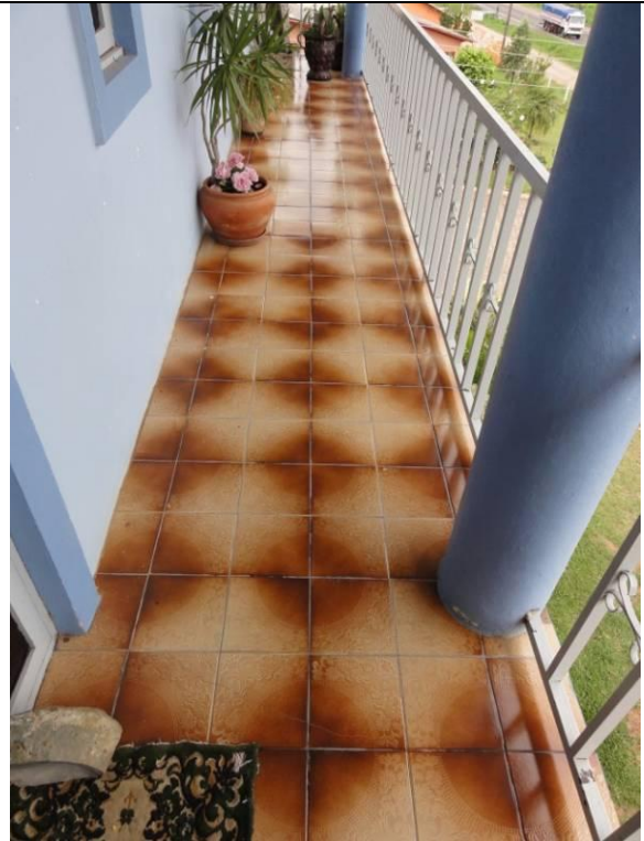
Piso superior – Sacada (DSC02323, 21/02/2011, 16:04h)
