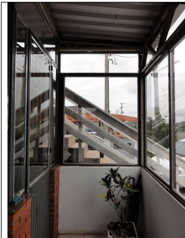
Piso inferior - Hall (DSC02803, 22/02/2011, 09:38h)
