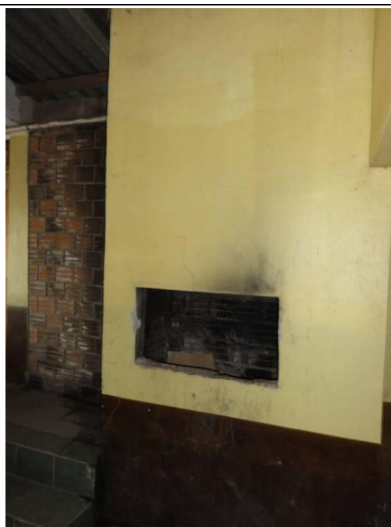
Piso superior (DSC03300, 22/02/2011, 17:09h)
