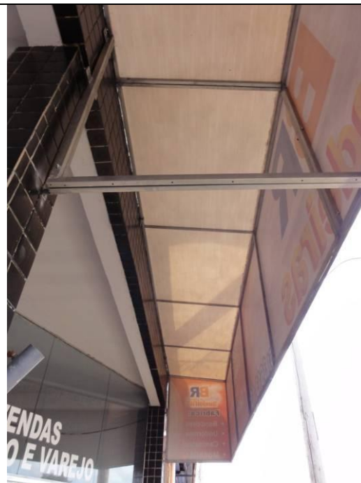
Fachada – Toldo (DSC03371, 23/02/2011, 08:55h)
