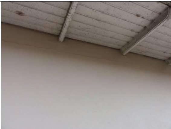
Piso superior – Sacada (DSC02942, 22/02/2011, 10:14h)
