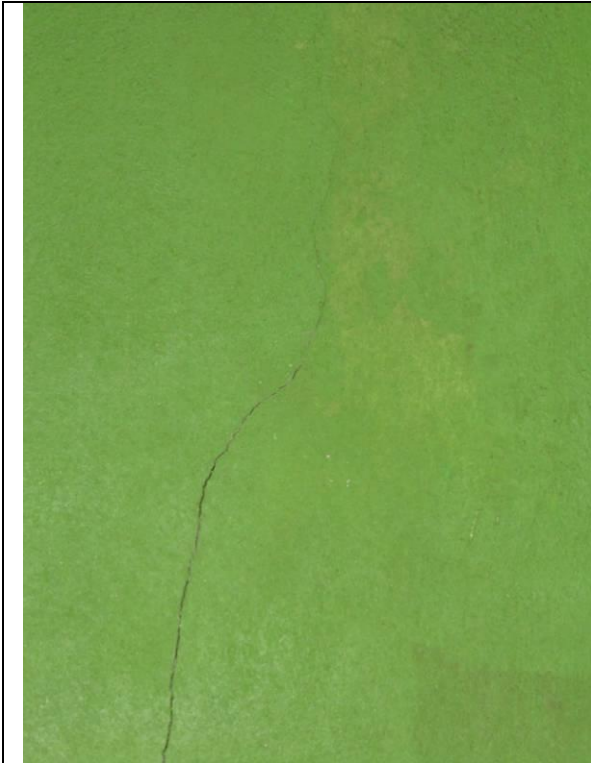
Piso superior - WC 2 (DSC02454, 21/02/2011, 16:35h)
