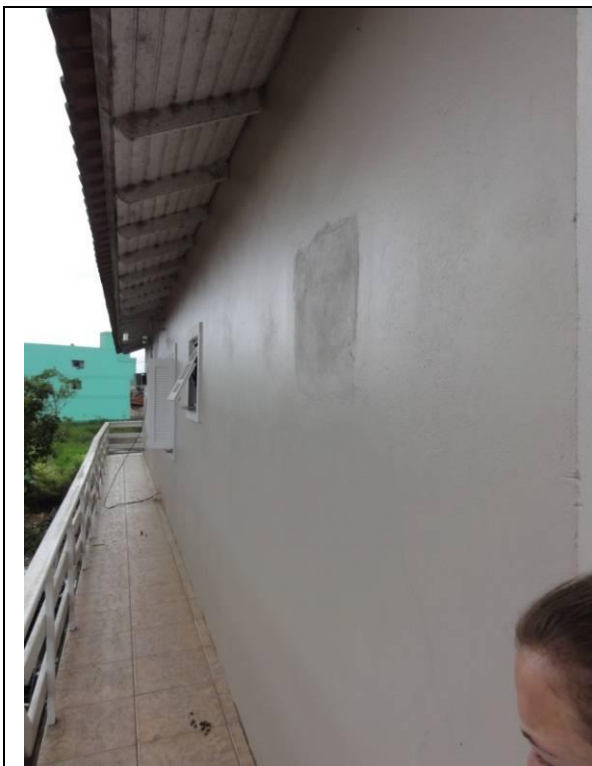
Piso superior – Sacada (DSC02938, 22/02/2011, 10:13h)
