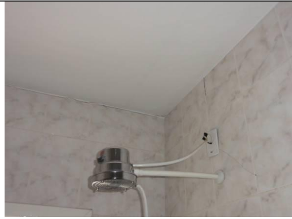
Piso superior – WC 1 (DSC02983, 22/02/2011, 10:21h)
