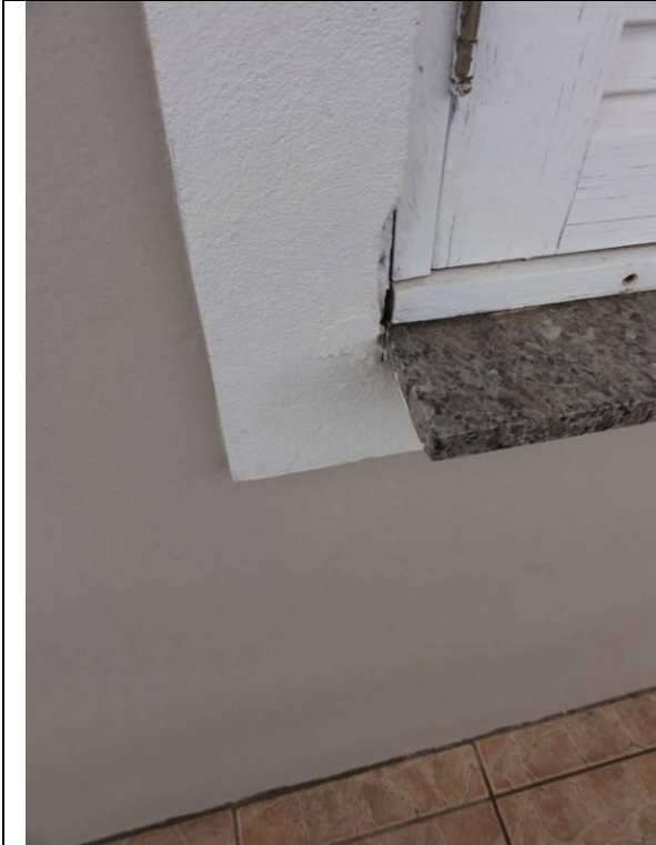
Piso superior – Sacada (DSC02952, 22/02/2011, 10:15h)
