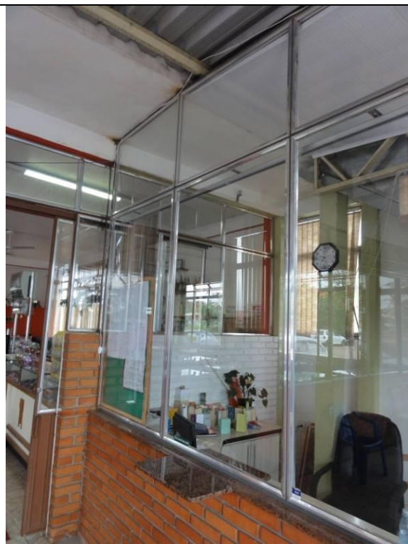
Piso inferior - Hall (DSC02804, 22/02/2011, 09:38h)
