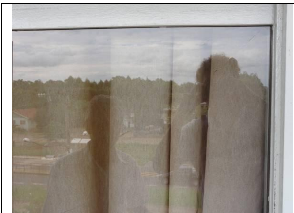
Piso superior – Janela (DSC02328, 21/02/2011, 16:05h)
