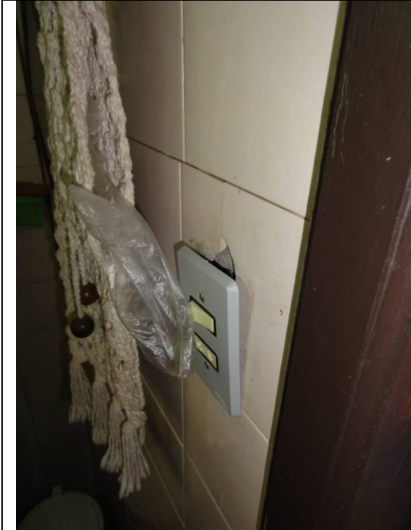
Piso superior - WC 2 (DSC02456, 21/02/2011, 16:35h)
