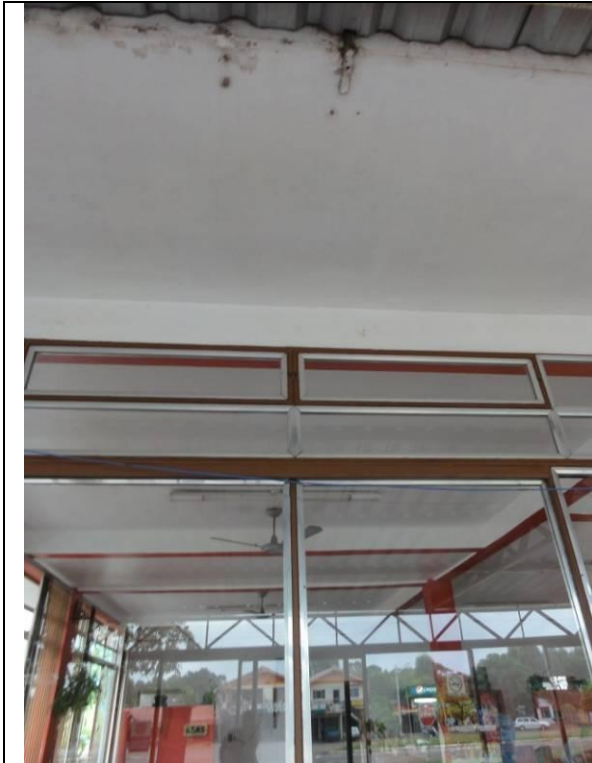
Piso inferior – Hall – Teto (DSC02811, 22/02/2011, 09:39h)
