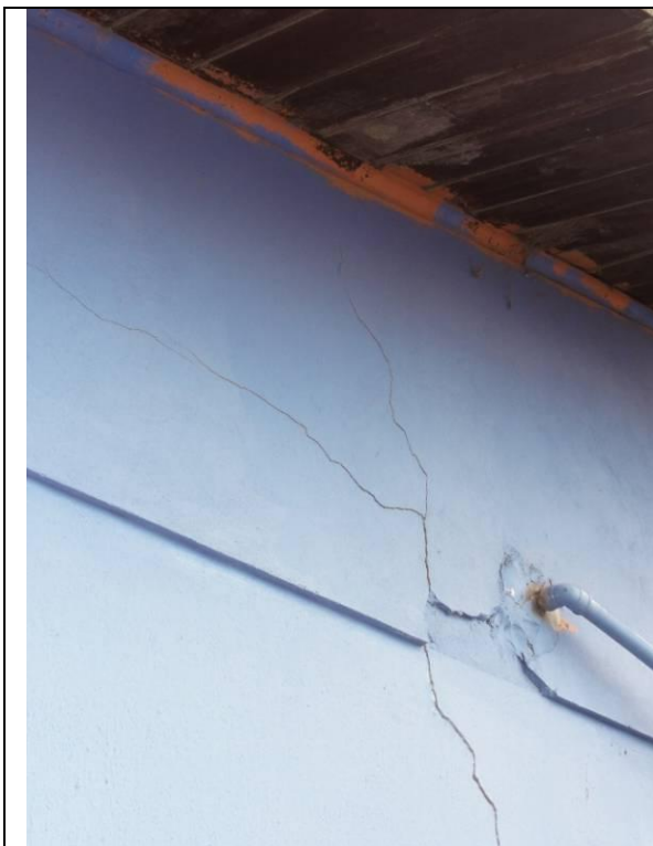
(Piso Superior - Sacada (DSC03574, 23/02/2011, 09:36h)
