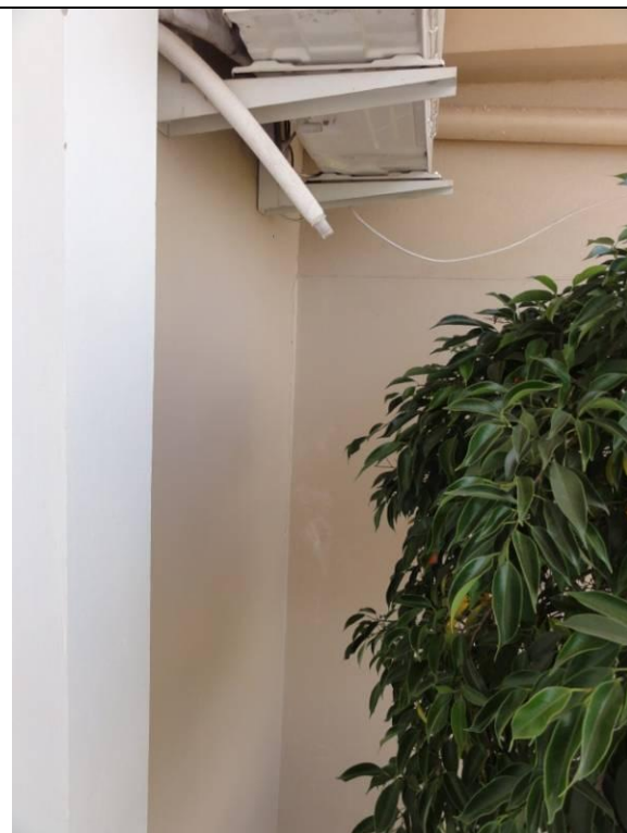
Piso superior - Sacada (DSC01023, 16/02/2011, 14:08h)
