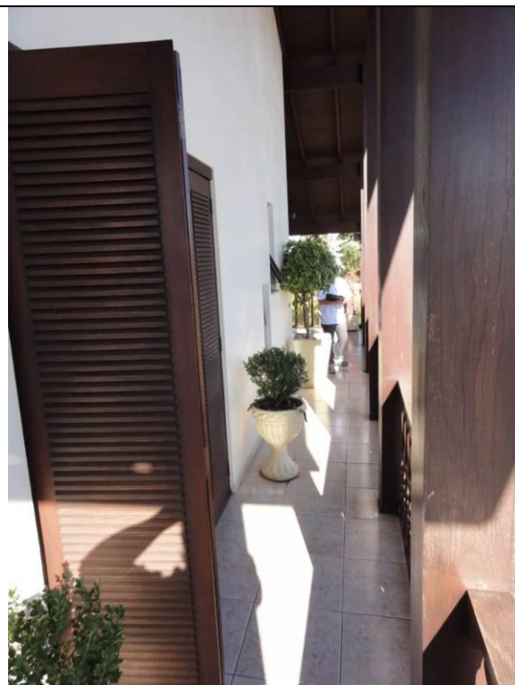
Piso superior – Casa – Sacada (DSC01240, 17/02/2011, 08:21h)
