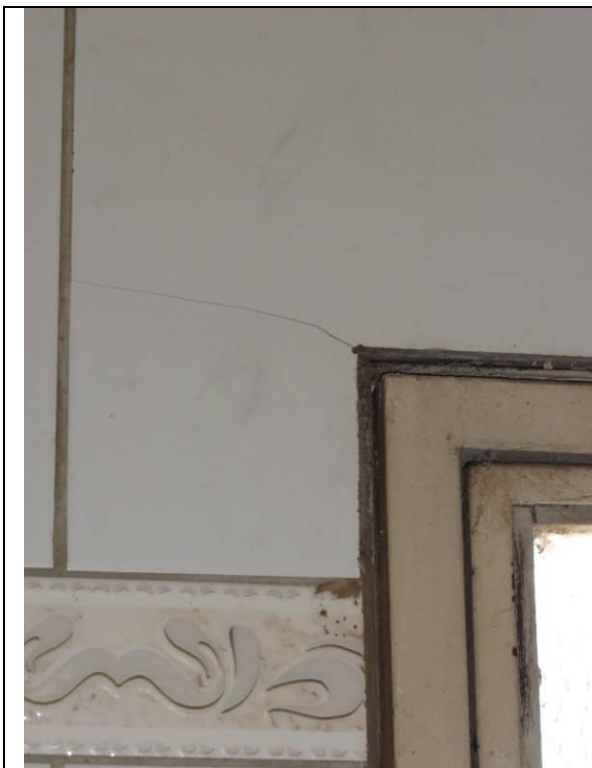
Piso inferior – Padaria (DSC01002, 16/02/2011, 14:03h)
