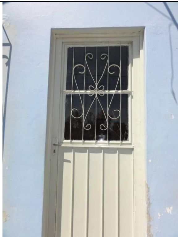
Fachada - Porta (DSC01488, 17/02/2011, 10:41h)
