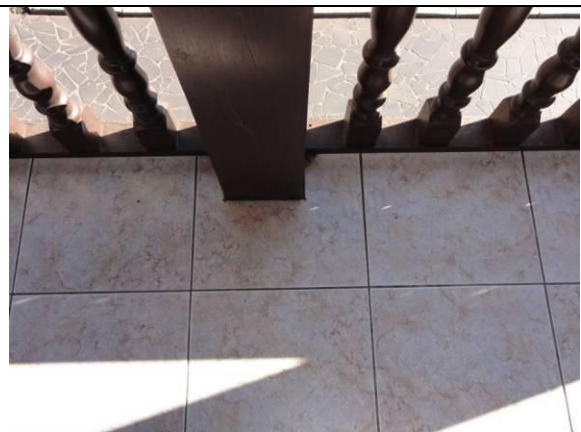
Piso superior – Casa – Sacada (DSC01244, 17/02/2011, 08:21h)
