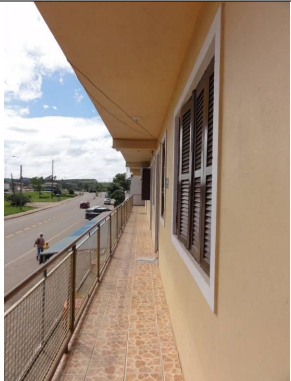
Piso superior – Sacada (DSC00865, 16/02/2011, 10:36h)
