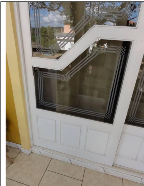
Sacada - Fundos (DSC01652, 17/02/2011, 15:51h)
