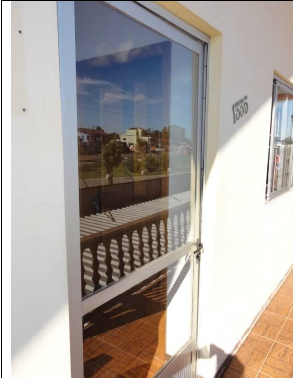
Piso superior – Parede A - Porta (DSC01331, 17/02/2011, 09:02h)
