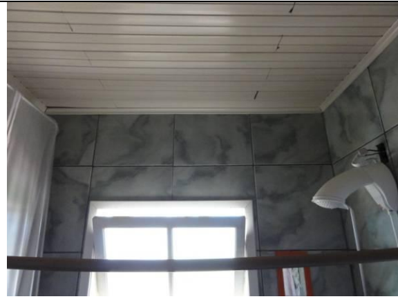
Quarto 3 – WC (DSC01637, 17/02/2011, 15:49h)
