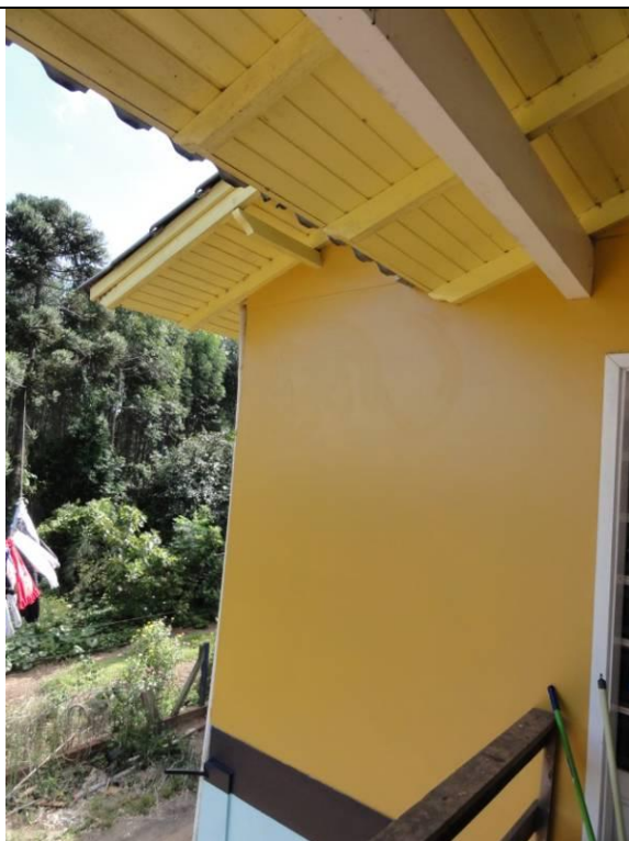
Sacada - fundos (DSC01676, 17/02/2011, 15:54h)
