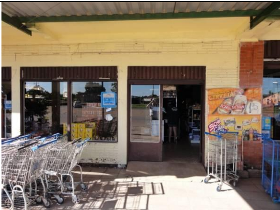
Fachada – Parede A (DSC01303, 17/02/2011, 08:53h)
