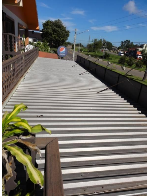
Piso superior – Vista sacada - Telhado (DSC01340, 17/02/2011, 09:05h)
