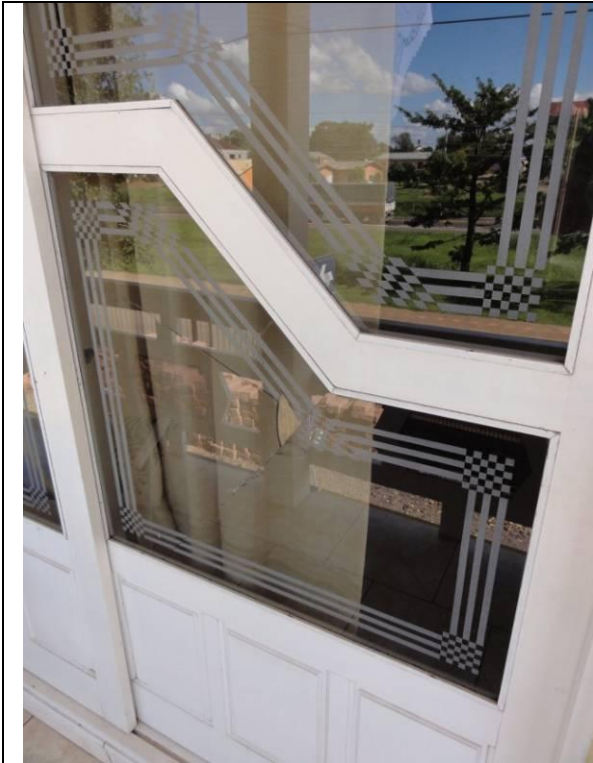
Sacada - Fundos (DSC01648, 17/02/2011, 15:51h)
