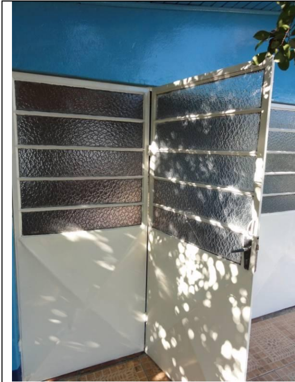
Fachada - Porta (DSC01256, 17/02/2011, 08:32h)
