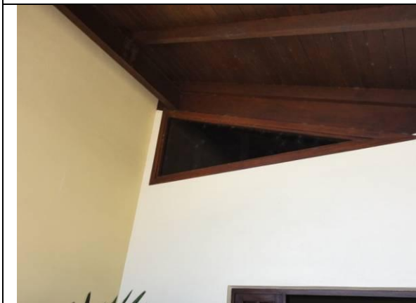
Piso superior – Casa – Sacada (DSC01243, 17/02/2011, 08:21h)
