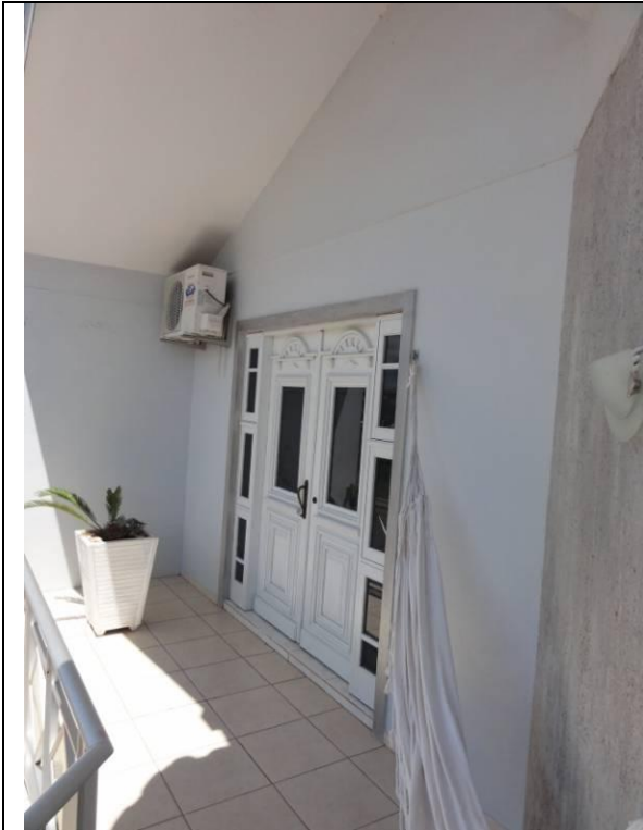
Piso superior – Sacada (DSC00941, 16/02/2011, 13:35h)
