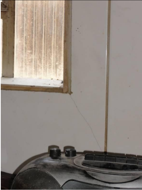
Piso inferior – Padaria (DSC01004, 16/02/2011, 14:03h)
