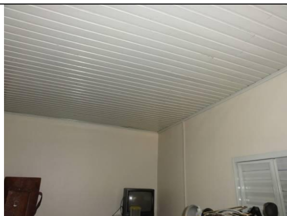
Sala – Teto com forro PVC (DSC01518, 17/02/2011, 10:46h)
