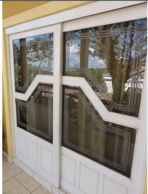
Sacada - Fundos (DSC01651, 17/02/2011, 15:51h)
