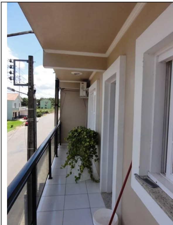
Piso superior - Sacada (DSC01016, 16/02/2011, 14:07h)
