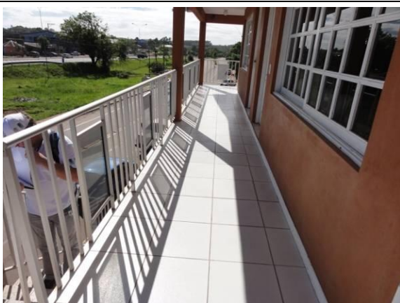
Piso superior – Sacada (DSC00672, 16/02/2011, 09:33h)
