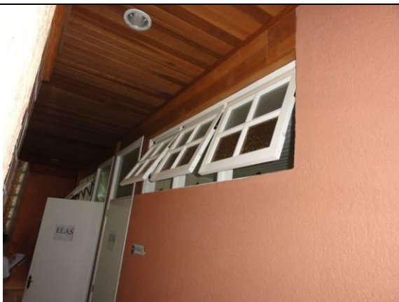
Corredor (DSC01920, 18/02/2011, 08:25h)
