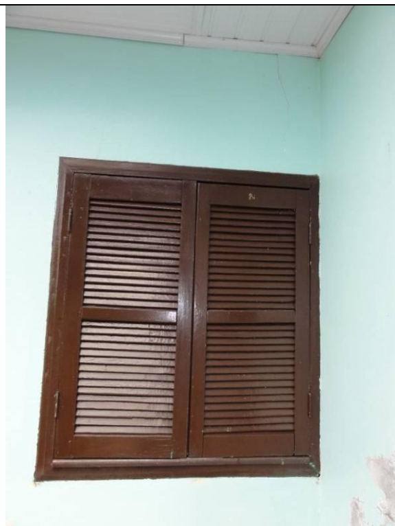
Janela – parede externa (DSC00109, 15/02/2011, 13:51h)
