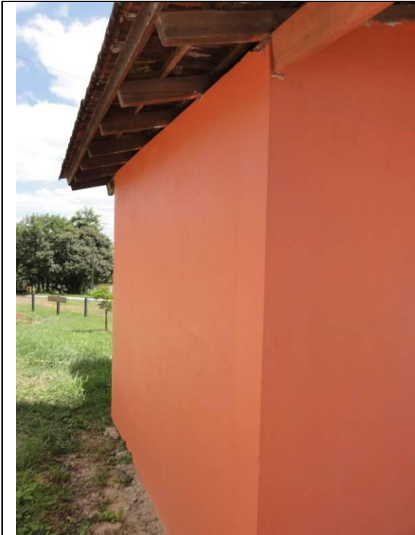
Parede D (DSC00200, 15/02/2011, 14:17h)
