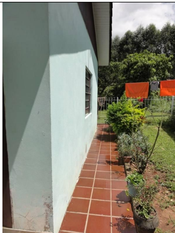
Parede B (DSC00075, 15/02/2011, 13:45h)
