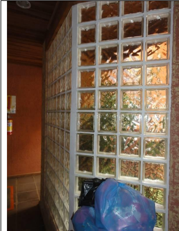
Corredor (DSC01926, 18/02/2011, 08:27h)
