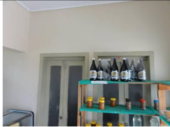
Parede interna (DSC00215, 15/02/2011, 14:20h)
