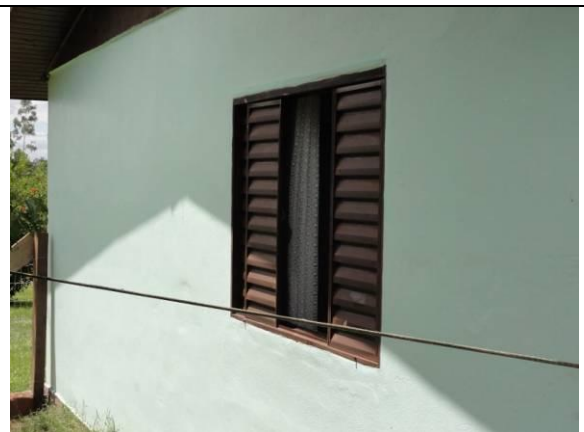
Lateral – parede B (DSC00019, 15/02/2011, 14:16h)
