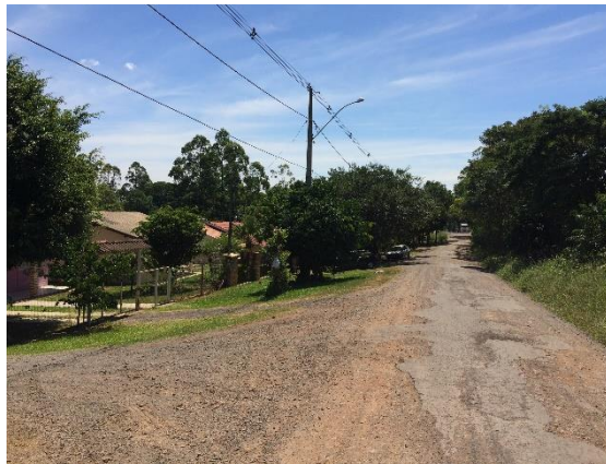
Figura 537 – Rua transversal a BR-386, Coxilha Velha, Triunfo/RS, Coord.: S29°41'56.58", W51°41'17.84".
