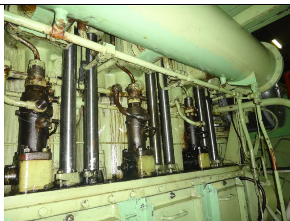
Aft Aux. Eng. Cyl#5 FO inlet line temp repair
