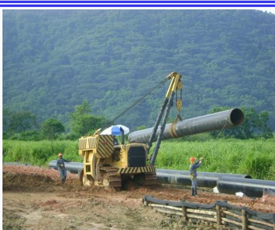
**Foto II.3-1 – Transporte de tubulação através do Side-boom.**
