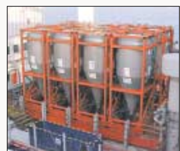
Drill cuttings are pumped from the CCB unit to ISO-PUMP storage tanks. Each ISO-PUMP unit stands on a weighframe to indicate load status.
