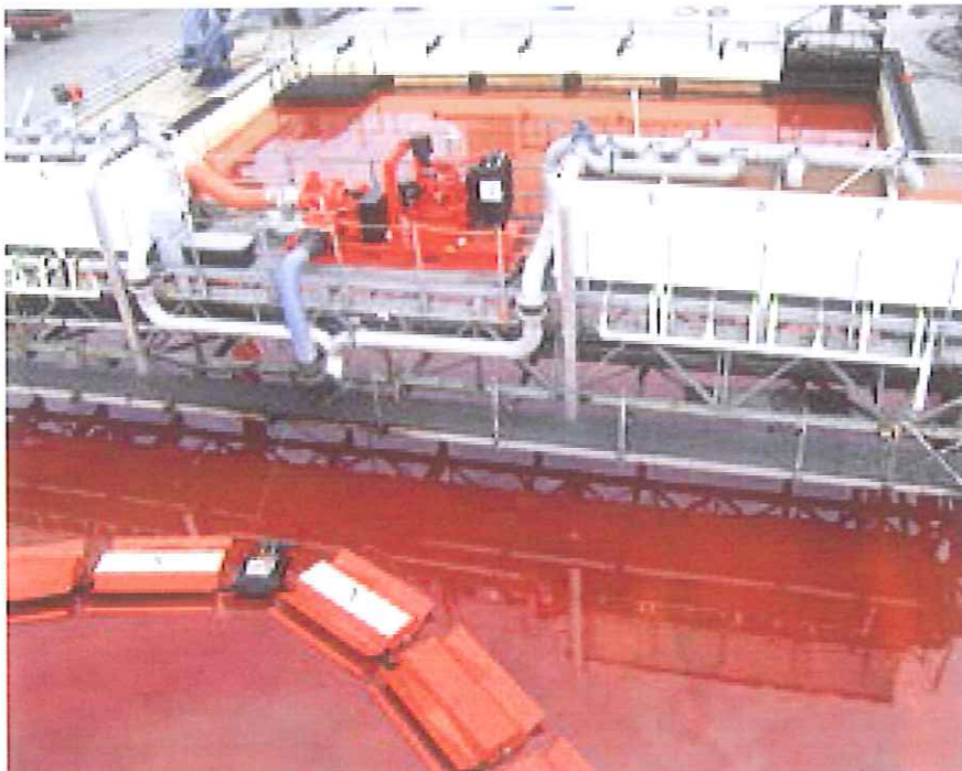
Figure 2 Recovery Tanks on the Auxiliary Bridge
