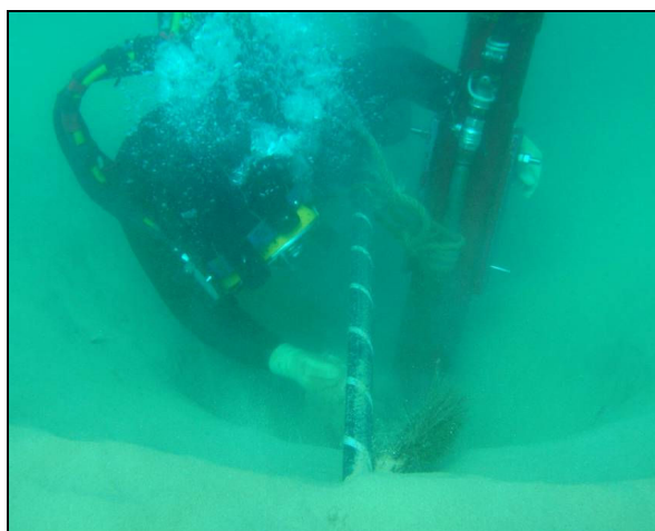
Figura III-12 - Ferramenta de jateamento manual - Airlifting
