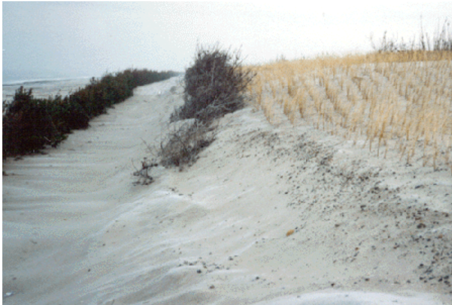
Figure 6.11 Planting of Marram grass and the placing of fences on artificial dunes (Danish Coastal Authority)
