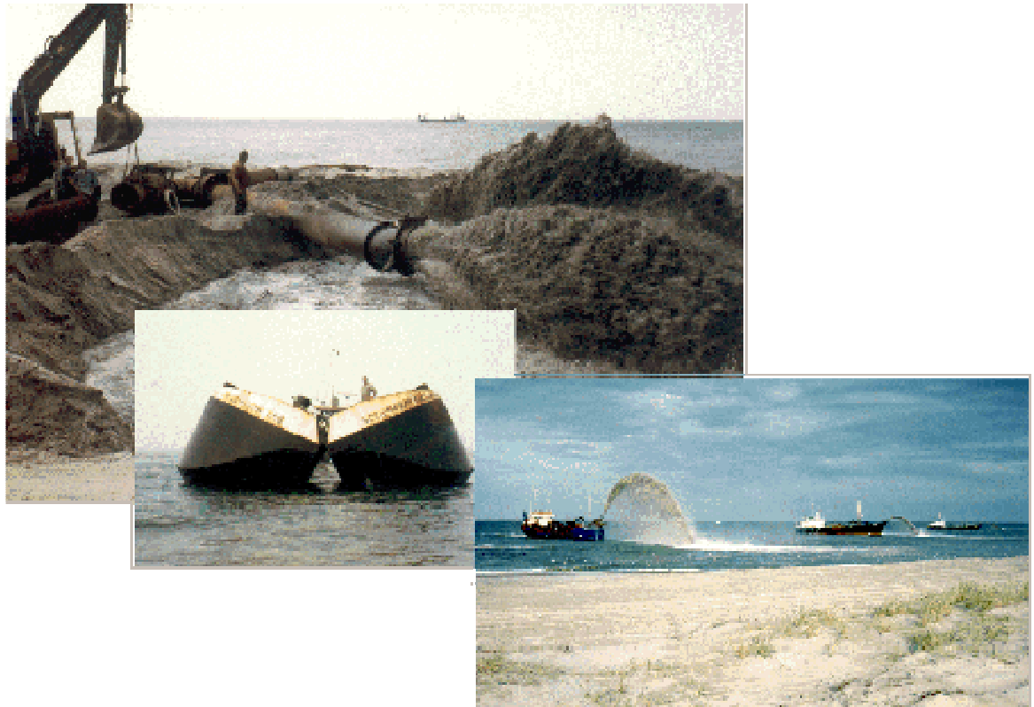
Figure 6.14 Nourishment methods in practice by the Danish Coastal Authority. Beach nourishment by pipe discharge on the beach and over the bow pumping and shoreface nourishment by split barge
