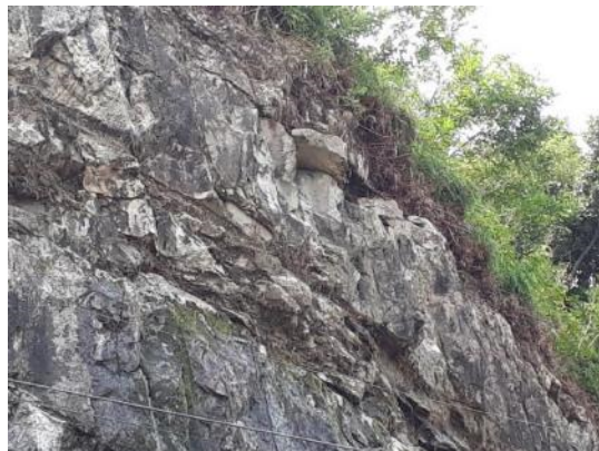
(b) Topo do talude
