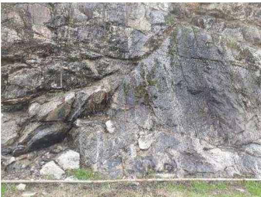
(a) Base do talude
