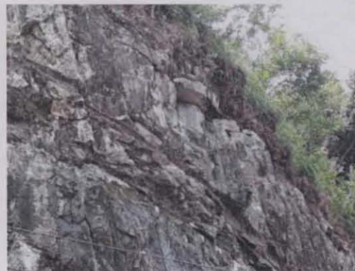
(b) Topo do talude
