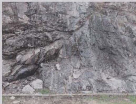
(a) Base do talude
