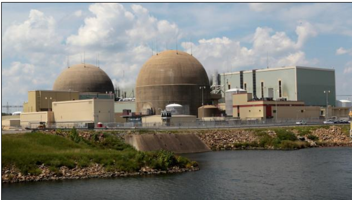
Figura 4-3 - Central Nuclear de Vogtle.
