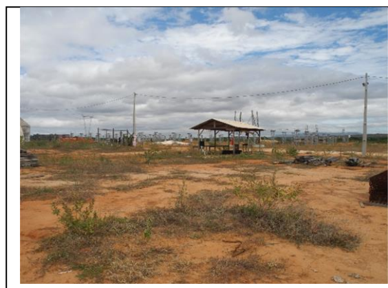
Foto 8.2.2-70 – SE Milagres II (P41, Milagres/CE). Coord. UTM 24S 508.405/9.188.394.
