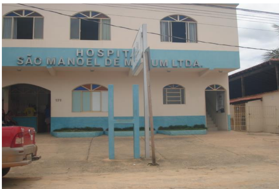
Figura 66 - Hospital Municipal São Manoel de Mutum
