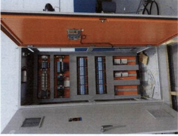
Detalhe painel de PLC
