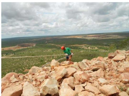
**Figura 11 – Decida no talude com EPI's (Petcon 2014)**
