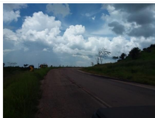
Figura 849 – Rodovia BR-163, Novo Progresso/PA (7,873934S; 55,182095W).
