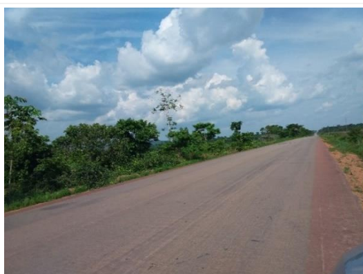
Figura 848 – Rodovia MT-419, Guarantã do Norte/MT (9,944856S; 54,987782W).
